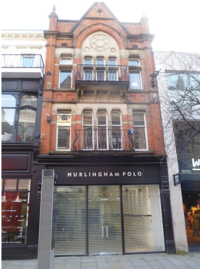
Figure 7.1 Frontage to 48 King Street in April 2024, Source: PBA Site Photograph.
