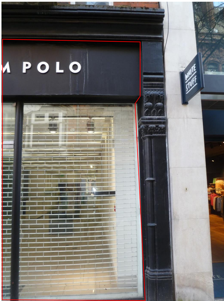
Figure 8.2 Inserted contemporary shopfront, identified in red
