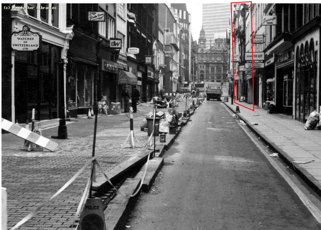
King Street, 1975, Manchester Archives, Application Property to Right of Picture
