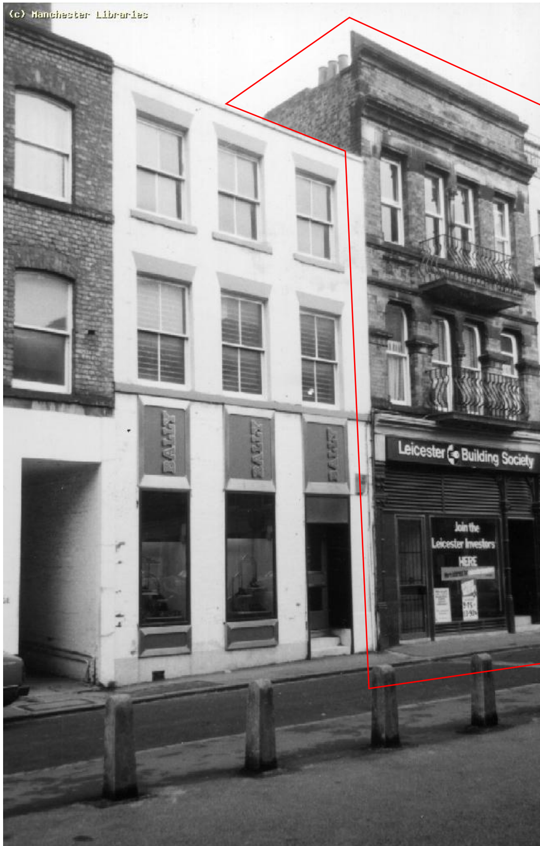
44 King Street, 1981, Manchester Archives, Application Property to Right of Picture
