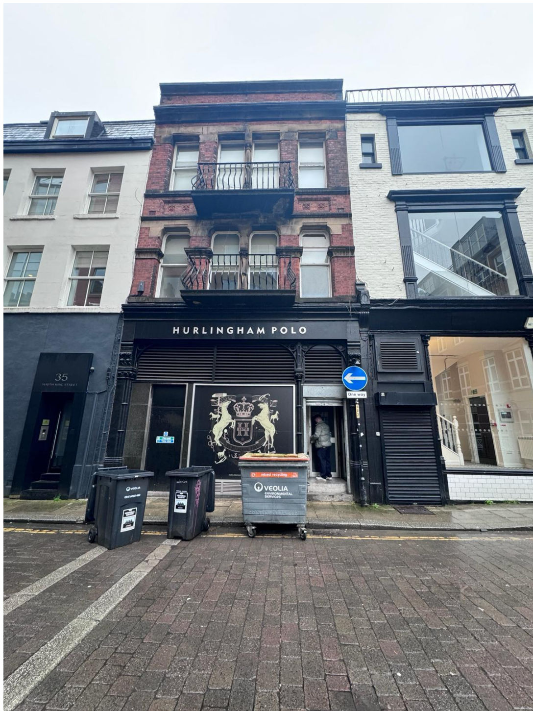
Figure 7.3 Unit viewed from King Street South in April 2024. Source: PBA Site Photograph.
