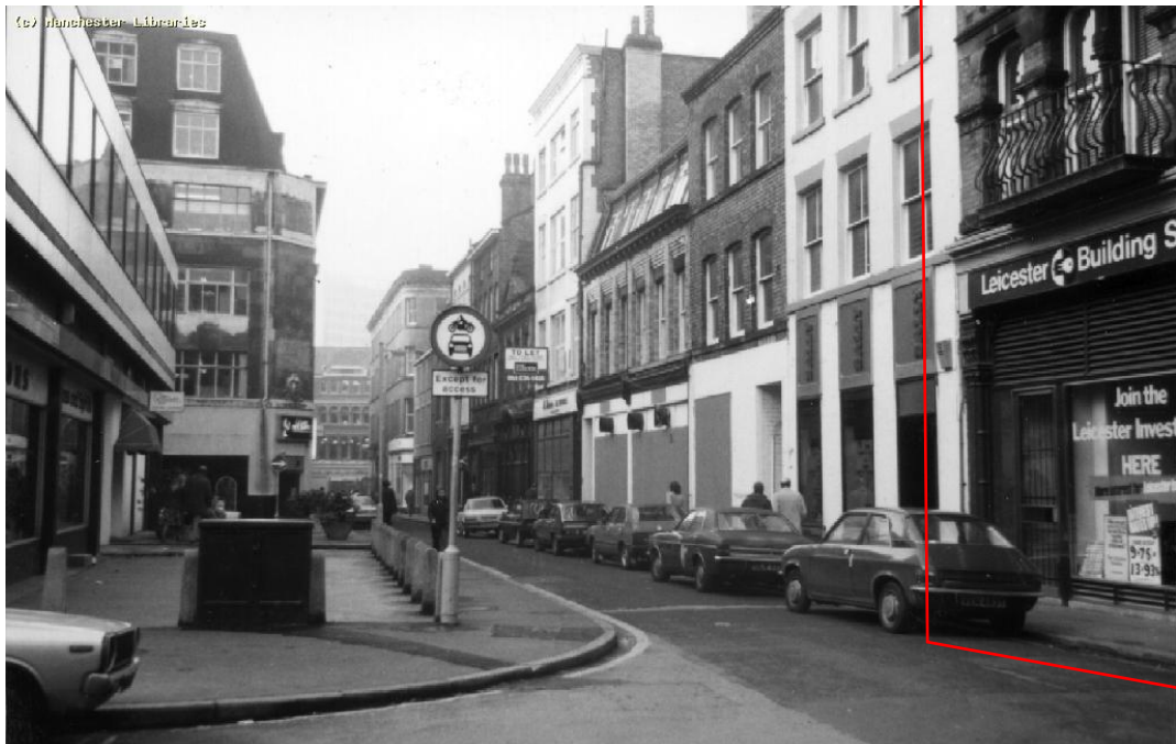
44 King Street, 1981, Manchester Archives, Application Property to Right of Picture
