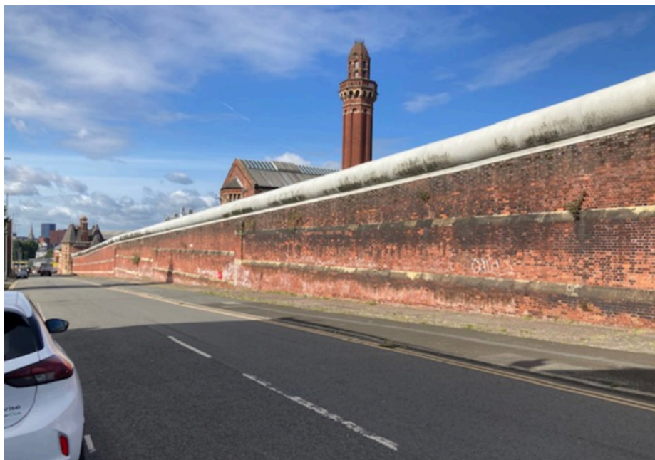
View of the ventilation tower from Southall Street
