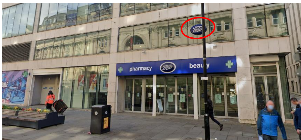
Figure 3: Boots signage at 32 Market Street (viewed from Cross Street) showing high level sign aligning with louvres
