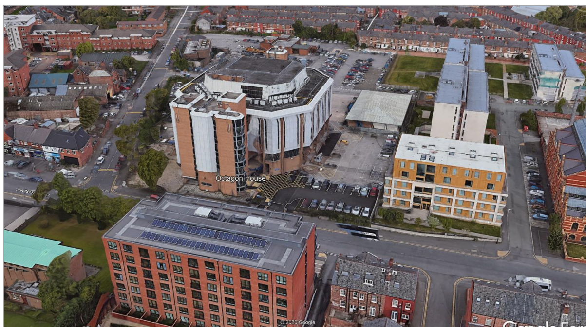
Figure 4: 3D imagery of existing buildings surrounding Octagon House (Google Earth 2020)
