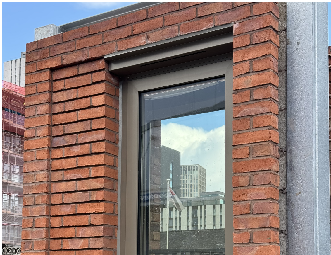
AS BUILT_TRICKLE VENT FLASHING MOCKUP (SITE PHOTO)
