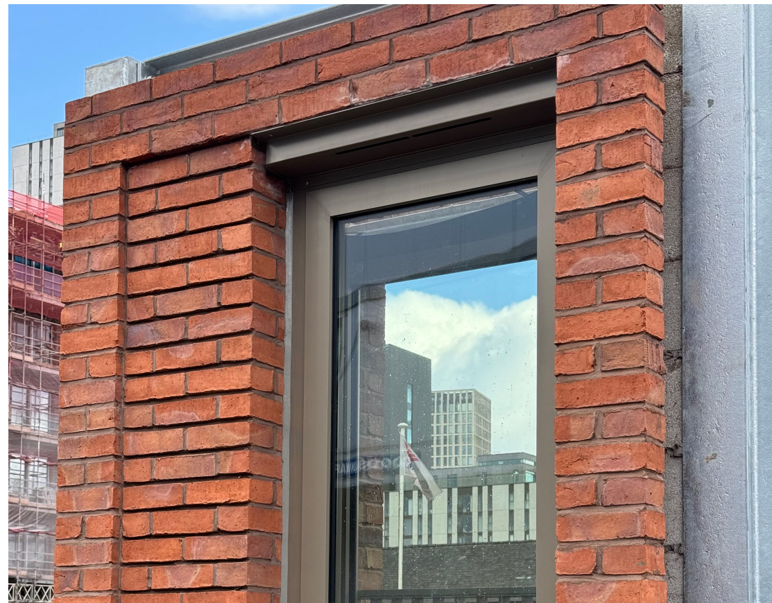
PROPOSED_TRICKLE VENT FLASHING MOCKUP (PHOTO MONTAGE)
