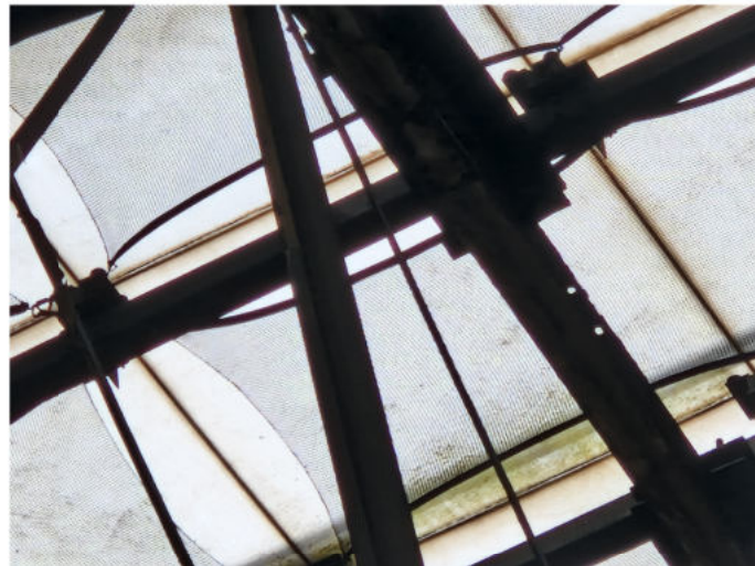
PHOTO OF EXISTING TRUSS No.11
