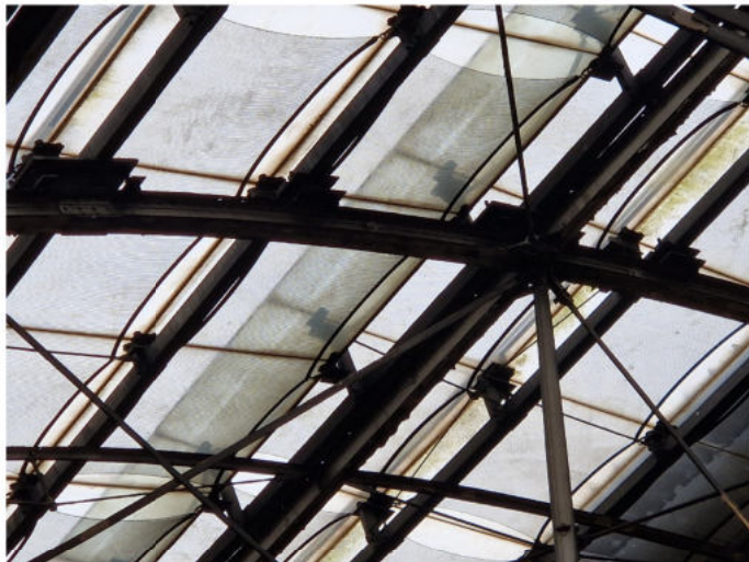
PHOTO OF EXISTING TRUSS No.11
