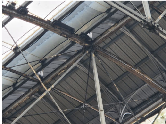
PHOTO OF EXISTING TRUSS No.11
