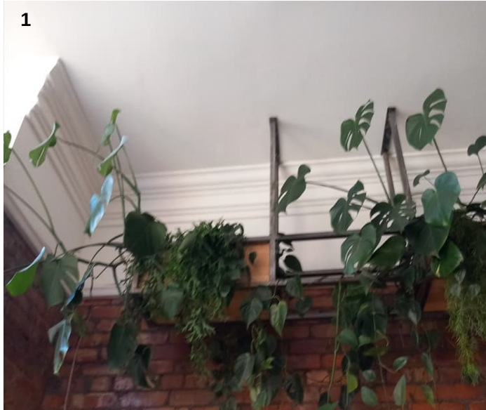
Plaster cornice and exposed brickwork
