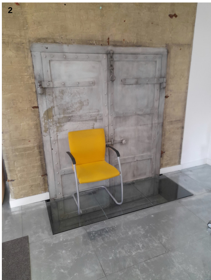
Exposed original lift doors and timber floor
