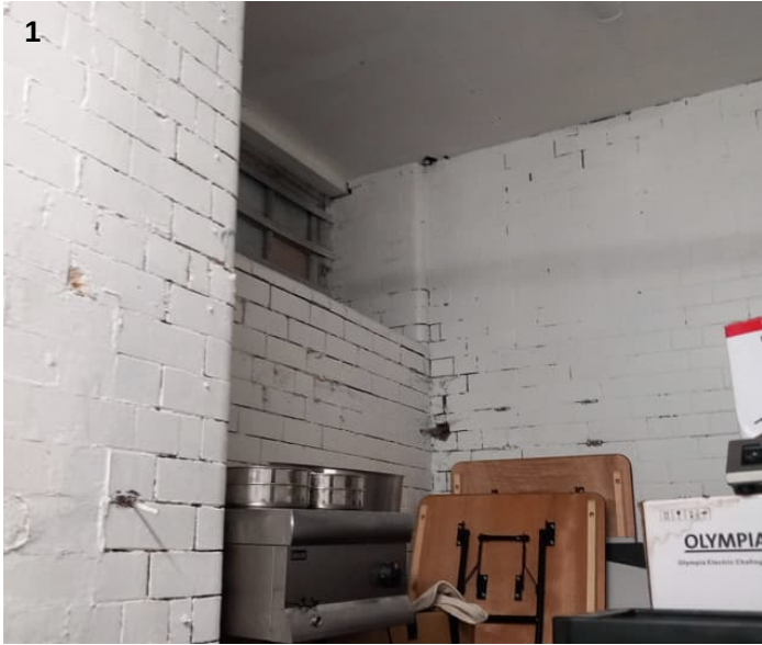
Painted glazed bricks
