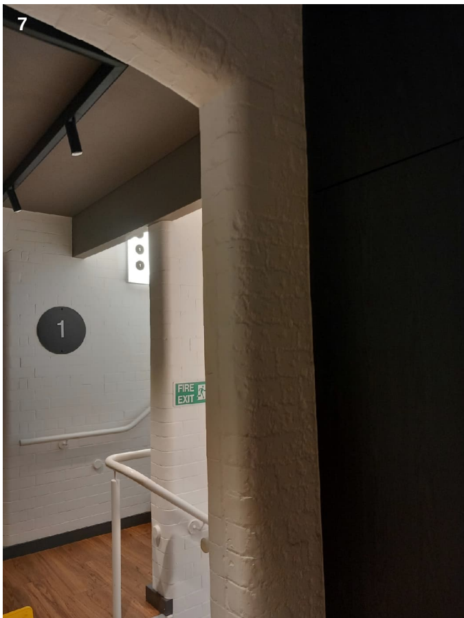
Exposed painted brickwork (common areas)
