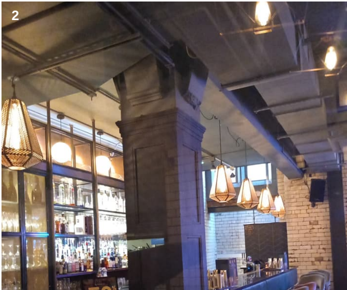
Decorative joinery/timber features to columns. Plaster downstands
