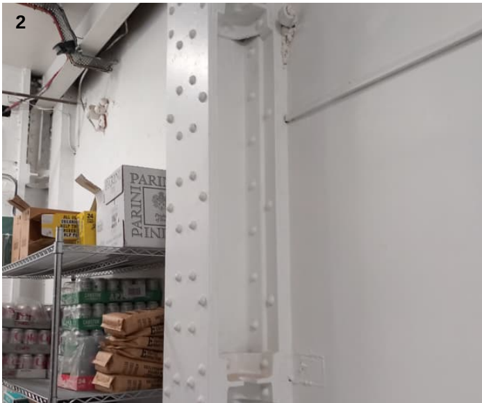
Painted steel columns
