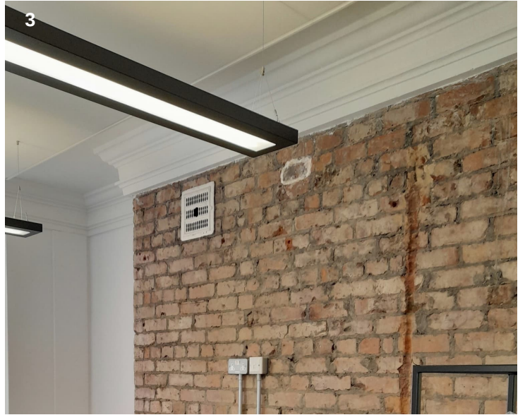
Plaster cornice and exposed brickwork
