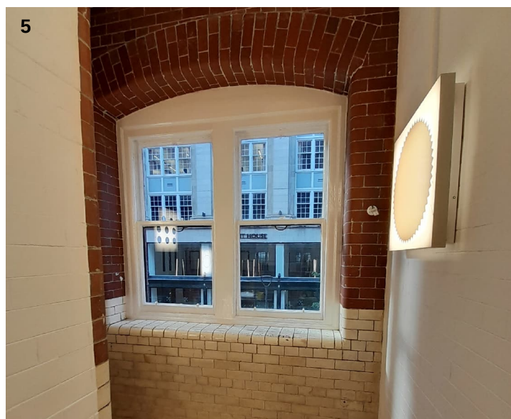
Exposed brickwork on half-landing between the ground and first floors
