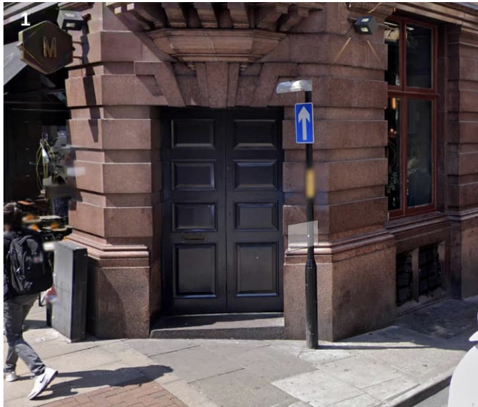
Timber doors to corner entrance (no.188)
