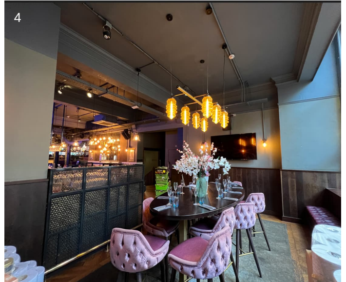
Plaster cornice and ceiling
