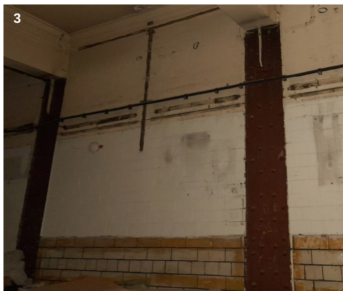
Exposed steel columns
