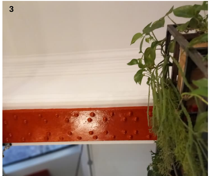
Exposed painted steel beam with decorative plaster details above
