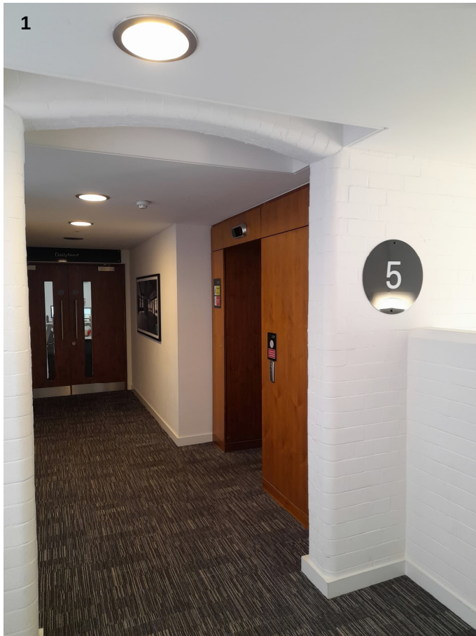
Exposed painted brickwork along corridor, including brick arch
