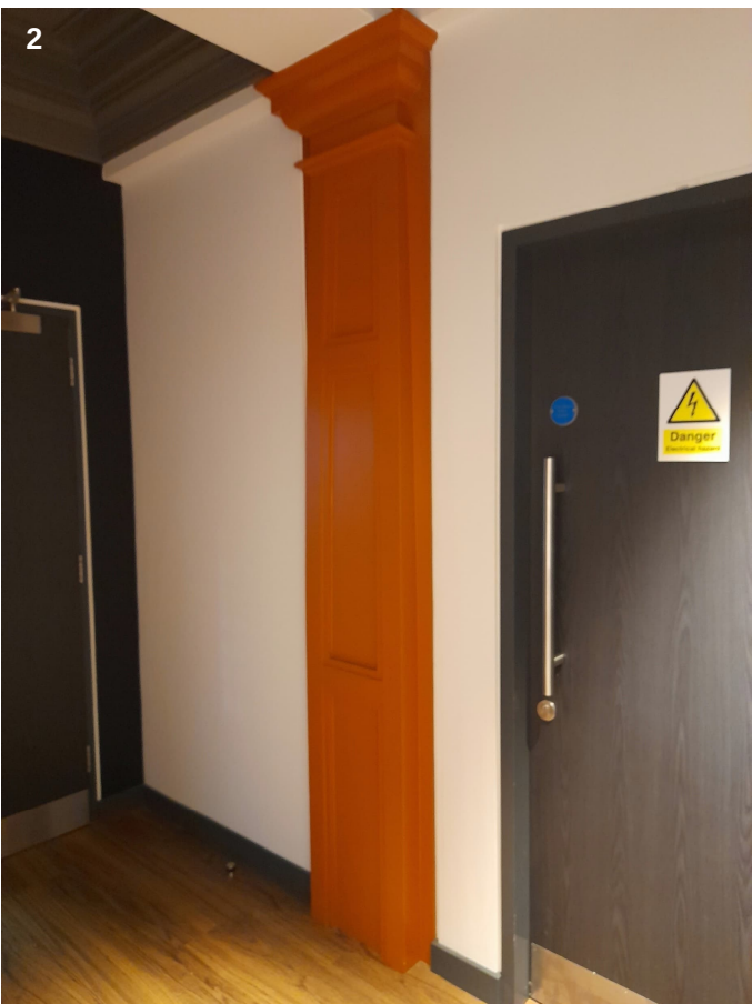
Pilaster along the corridor leading to the main staircase
