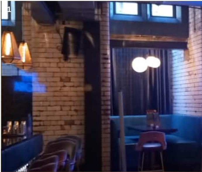
Glazed bricks to wall
