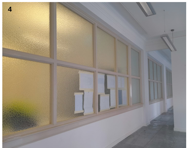
Timber screens and plaster cornices
