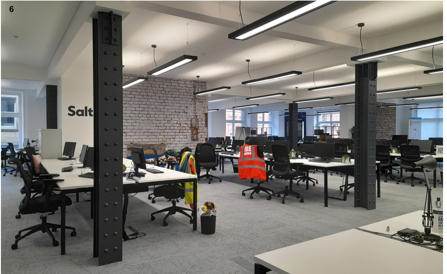
Exposed painted steel columns and exposed brickwork
