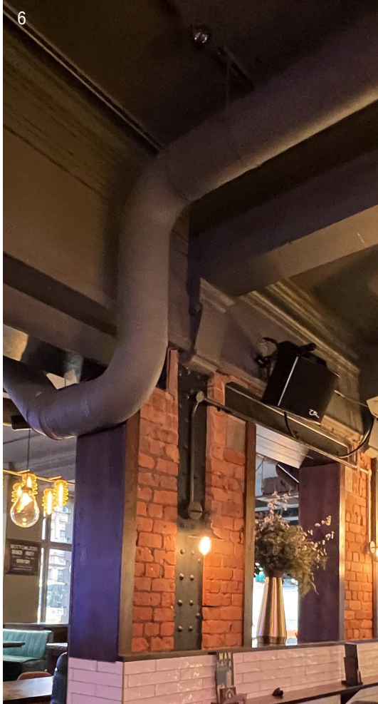
Plaster Cornice, downstand and ceiling.
