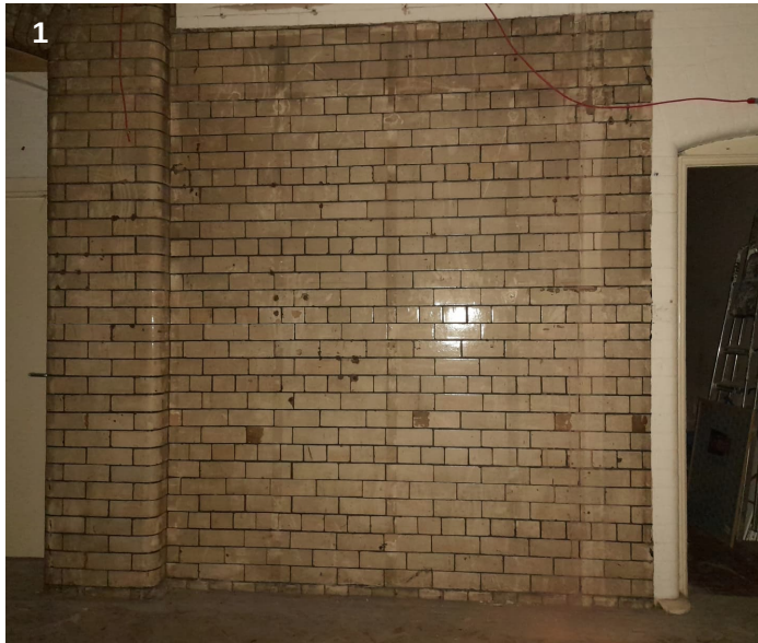
Glazed bricks to wall
