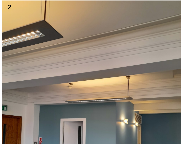
Plaster cornice in office area
