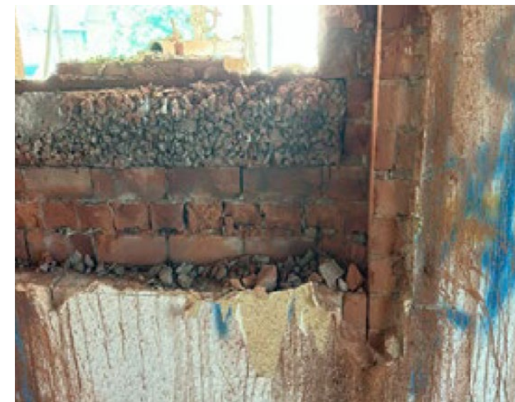
Other elements of brick are poor in appearance, with a patchwork of pieced together brick types, which is aesthetically poor. In situ concrete cills are exposed externally, (internal photograph below).
