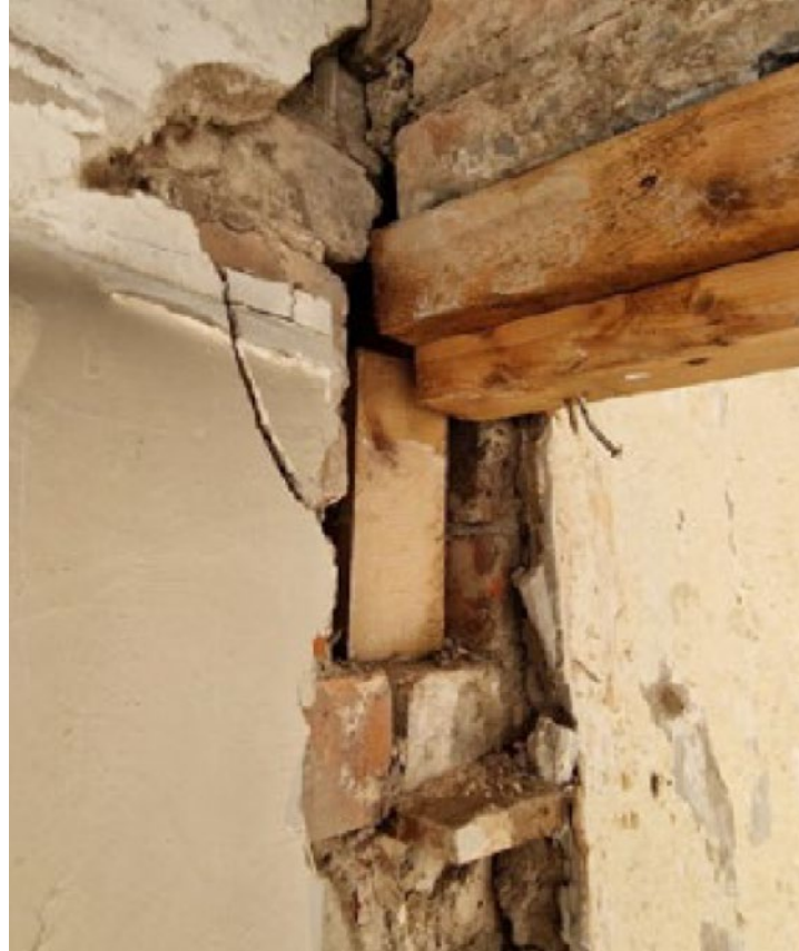
External brickwork has historically been removed to allow for internal wall support modification, as seen in the photo above and below. The exposed timber joists were then masked in the concrete.
