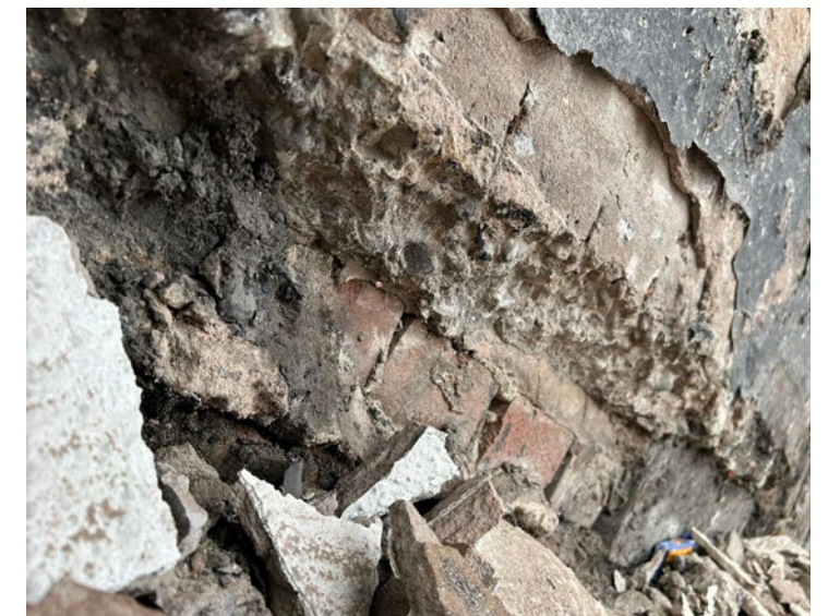
The patchwork of brick has been rendered with a mixture of adhesive and concrete to cover over its lack of unity. This process has led to damp and non-breathable sections of brickwork. The brick is therefore irreparable.
