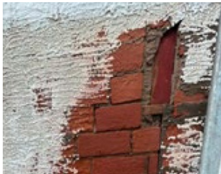
External brickwork has historically been removed to allow for internal wall support modification, as seen in the photo above and below. The exposed timber joists were then masked in the concrete.
