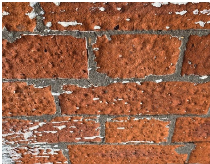
Concrete applied to the face of the brick across the entire structure. This has proven extremely difficult to remove completely, and where removed in section has defaced the existing brick.
