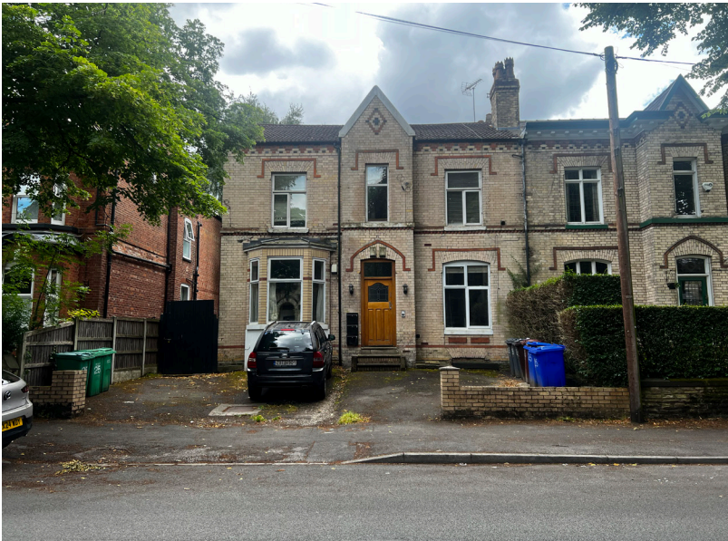
25 Mayfield Road viewed from the front
