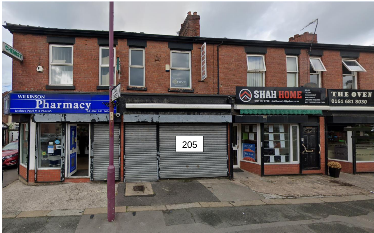
Photograph showing the application site and adjoining commercial properties
