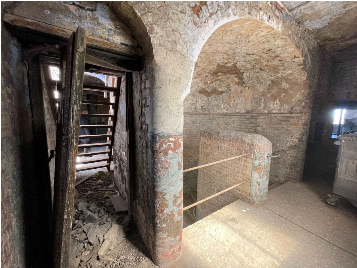
The landing of the east staircase at 6 th floor level, showing the original plastered domed ceiling of the staircase, which will be retained as part of the paint removal process.
