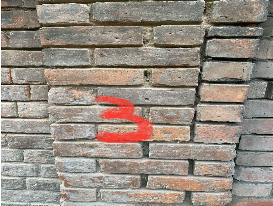
Photo 3 - Raked out cutting through the centre of the mortar with a thin blade and then taken out the mortar using handheld tools to the required depth and brushed out leaving the area clean.
