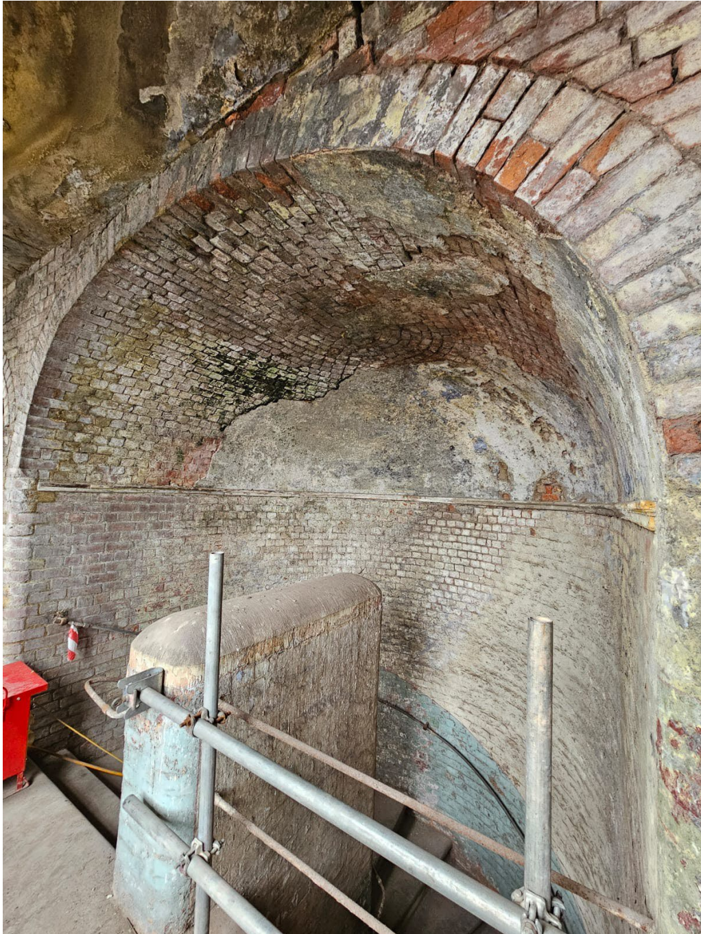
The landing of the west staircase at 6 th floor level, showing the remains of the original plastered domed ceiling of the staircase, which will be retained as part of the paint removal process.
