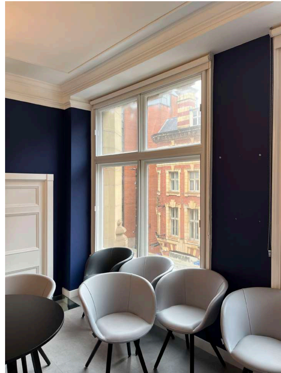
Typical Secondary Glazing previously installed to lower floors
