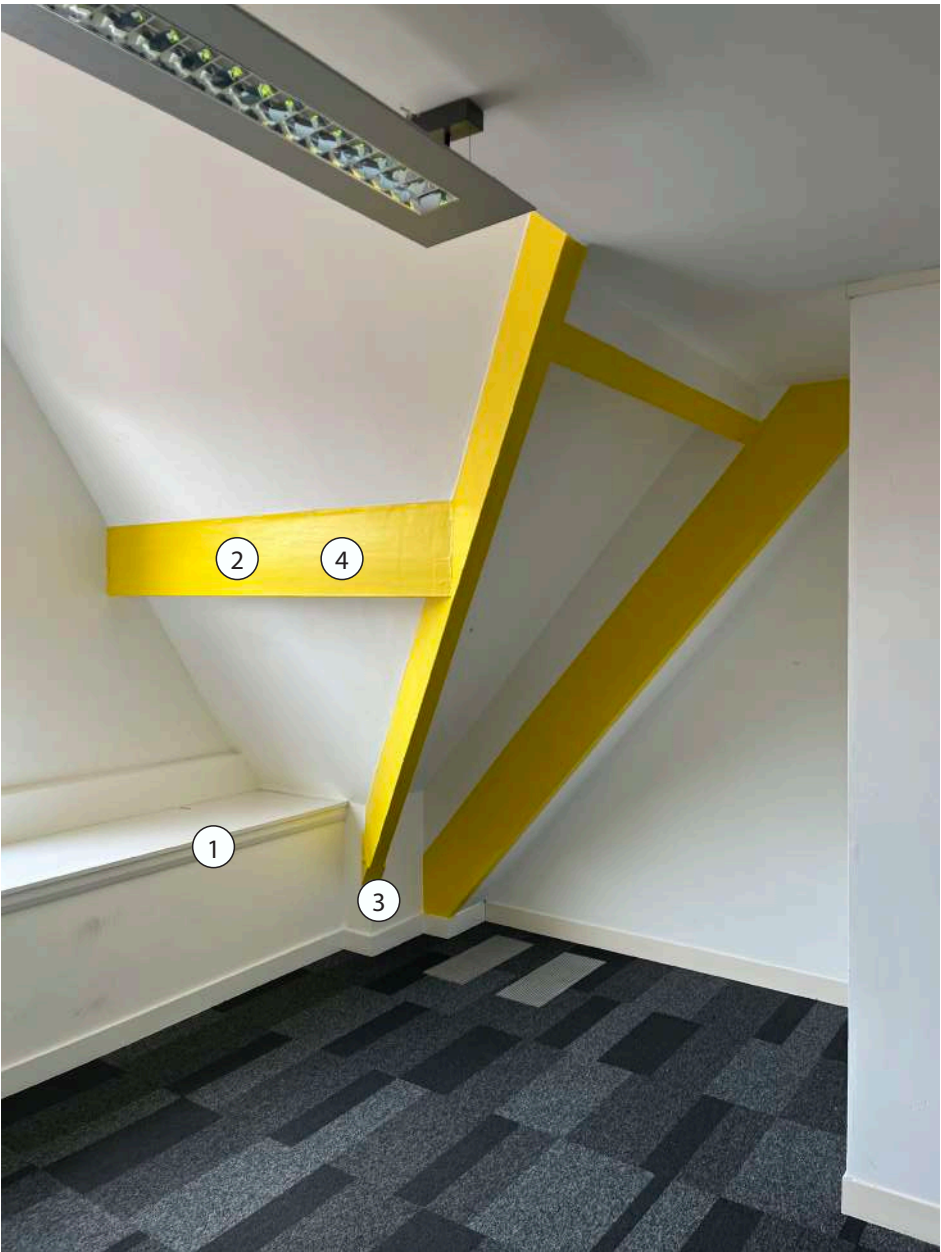
Typical Existing Raked Ceiling
