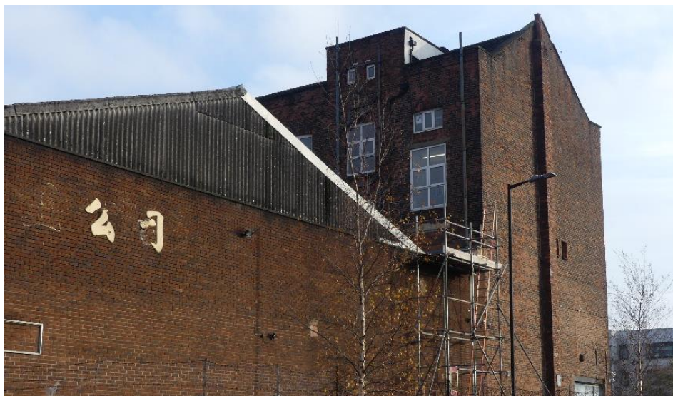
Figure 1.11: The southern part of the application site, including the southern stairwell projecting above the adjoining supermarket
