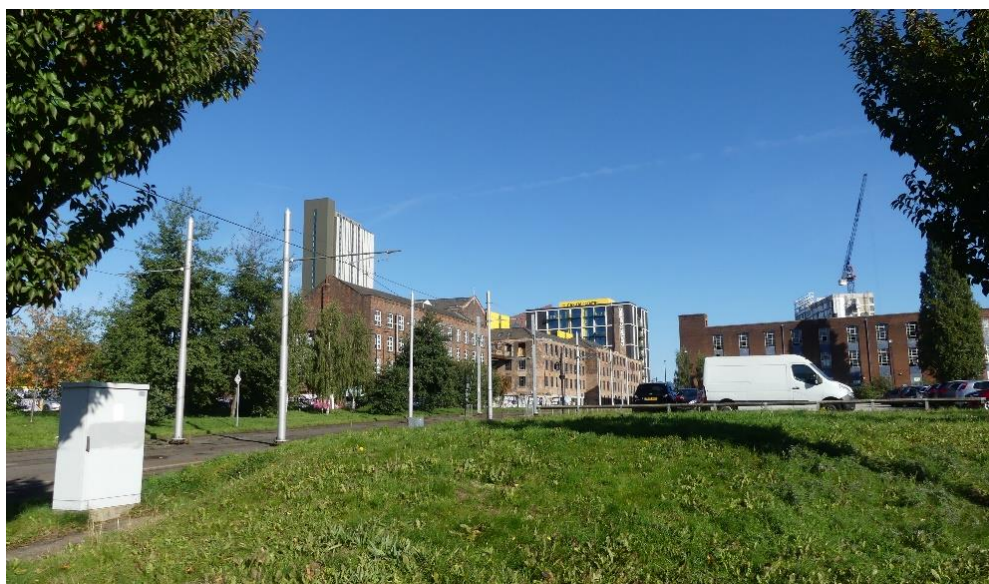
Figure 1.17: The view northwards towards the application site from Sheffield Street
