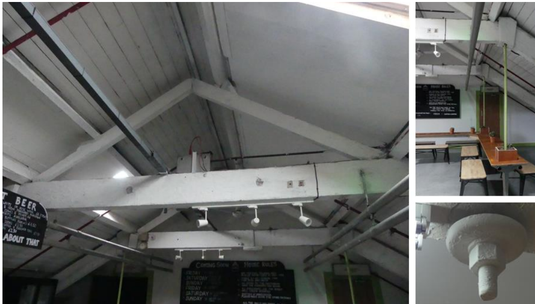
Figure 1.14: The interior of the roof and detail of the tie rods that are fastened through the floor beams
