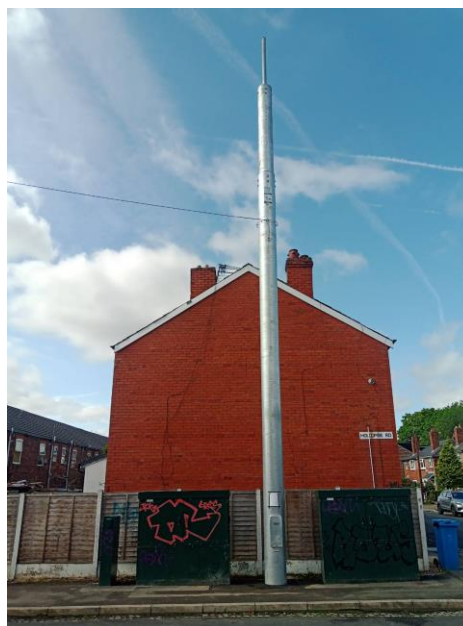
Figure 1: Photograph of the existing pole
