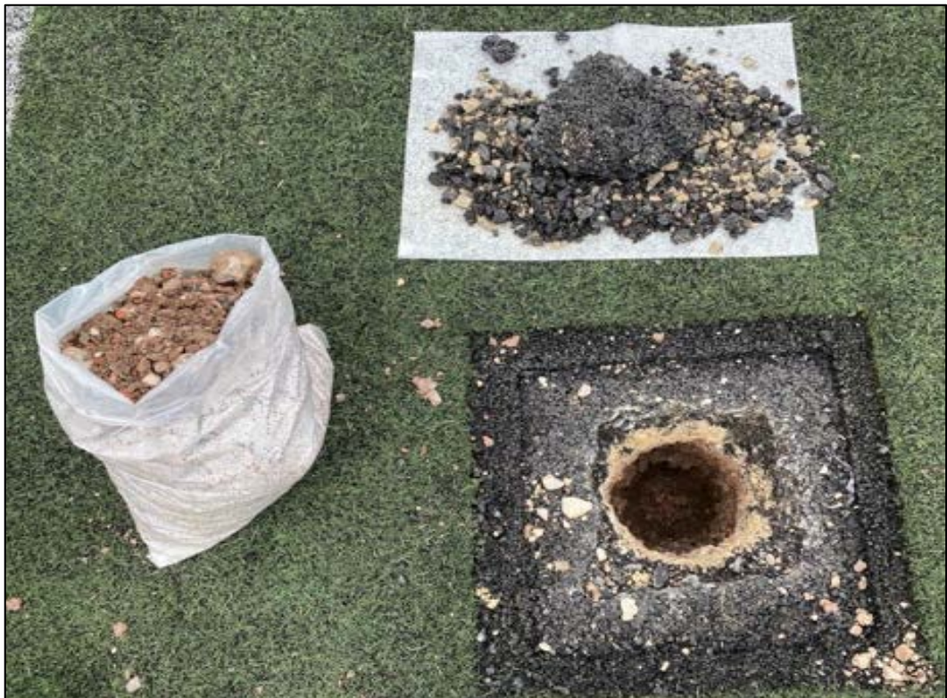
Figure 4-3: HP09 at completed depth showing Made Ground subgrade
