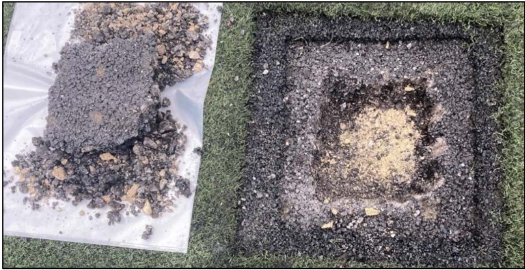
Figure 4-2: Asphalt onto granular subbase in HP14
