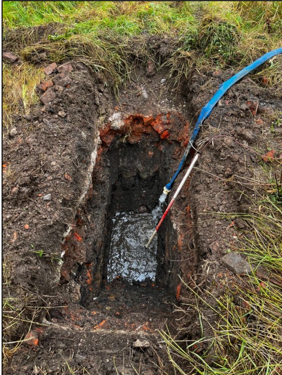
TP1 filling operation
