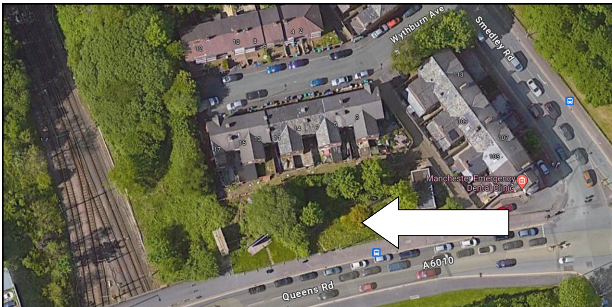
Application site indicated by arrow (extract Google Maps)
