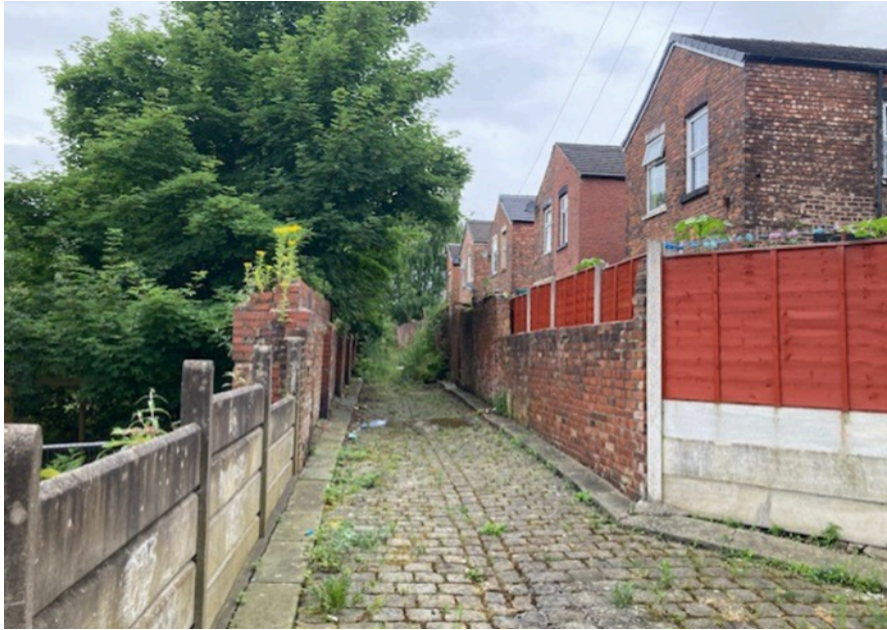
View of rear alleyway bounding the site to the rear (left) and facing residential properties along Wythburn Avenue (right)
