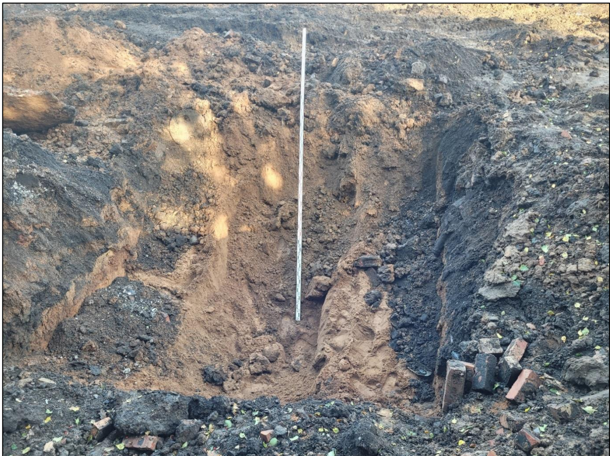
Figure 9: Photograph of Tank Trial Pit, Post Tank Removal
