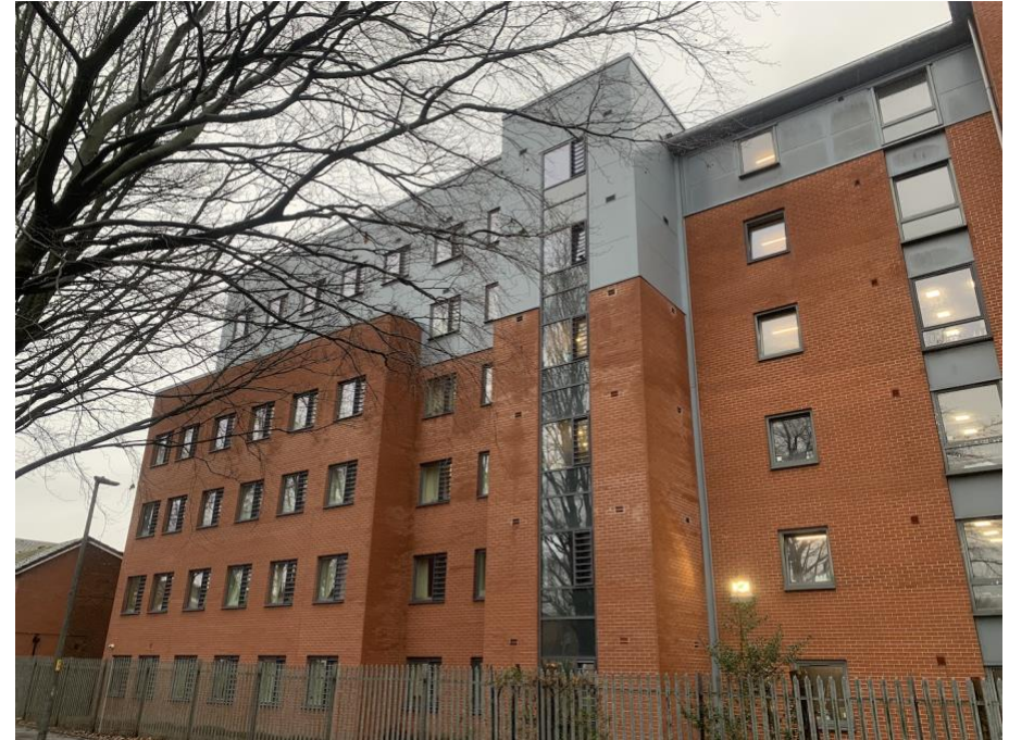
View along the side elevation from Kincardine Road.
