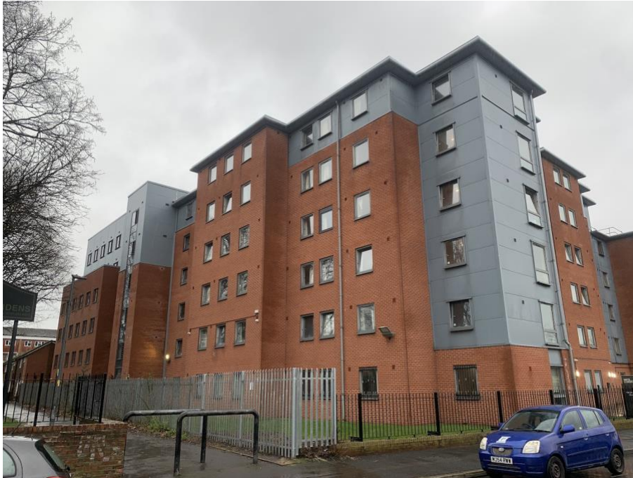
View along the side elevation facing Gartside Gardens from Kincardine Road.
