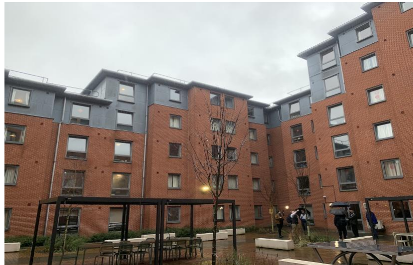
View of existing block from within the courtyard – 2.
