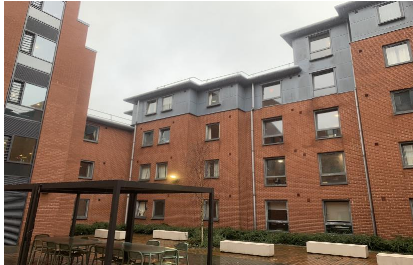
View of existing block from within the courtyard - 1.
