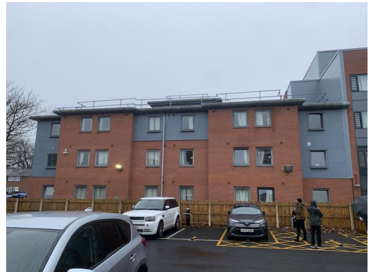
View to rear elevation from the Car park to rear of the property.
