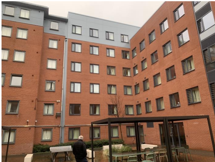
View of Kincardine existing to new build block from within the Courtyard.
