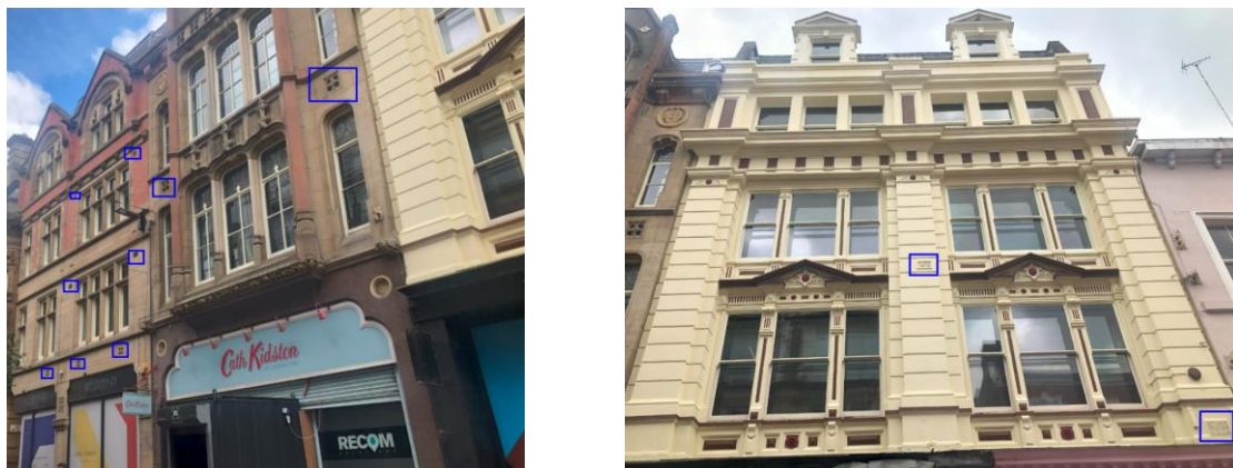
Figure 2 Photograph showing visible MVHR terminations at position 'X'
