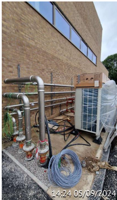
Figure 4: Air Source Heat Pump Installation
