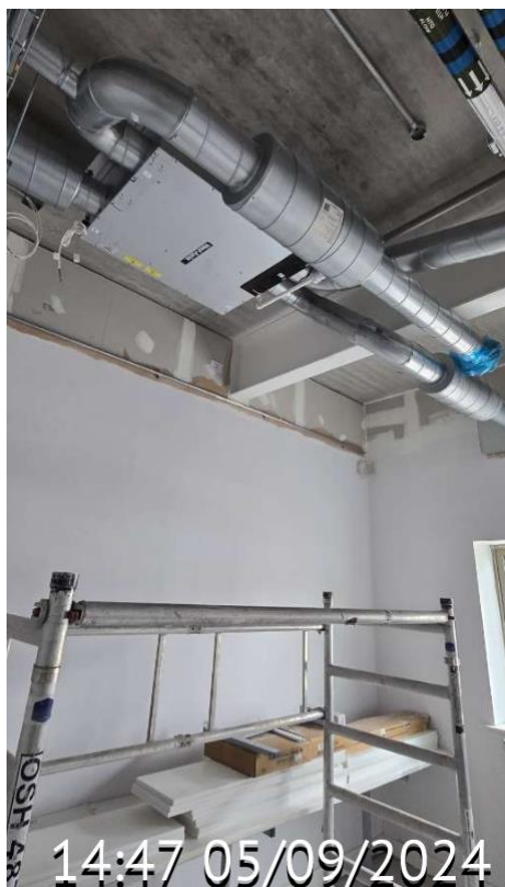
Figure 5: Mechanical Ventilation with Heat Recovery (MVHR)
