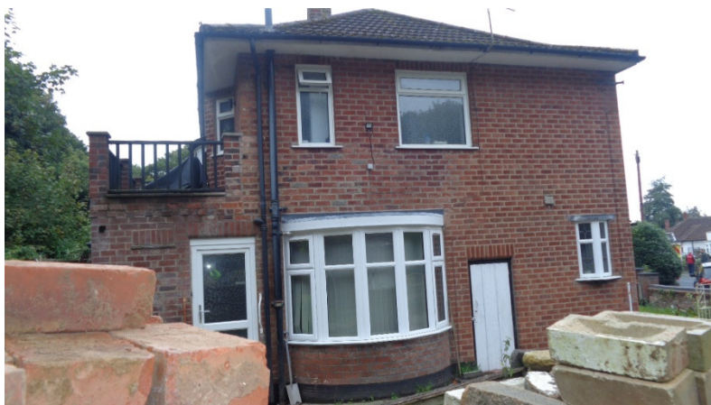
Gable of Adjacent Property Nr 48.
