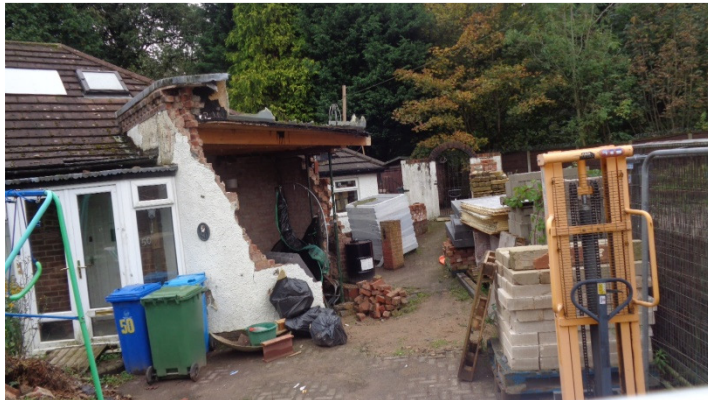
Front Elevation to Application Property.
