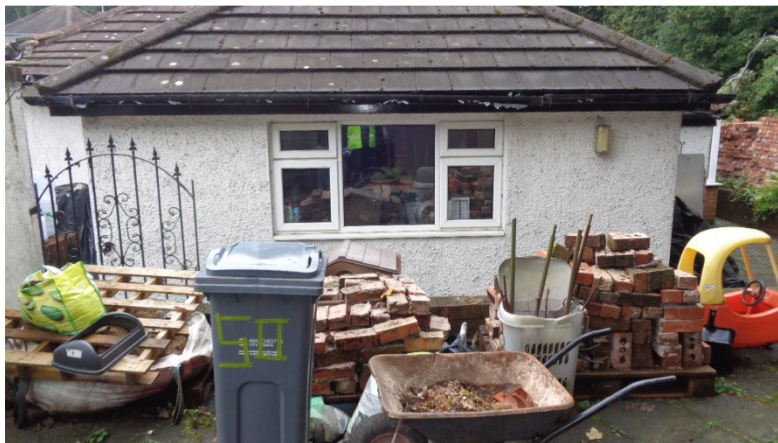
Gable Elevation of Application Property facing Proposed Garage Location.
