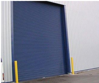
3.7 (A) Operational Door – Level access, sectional, insulated door Plastisol Coated Finish in Midnight Blue (RAL 5003)
