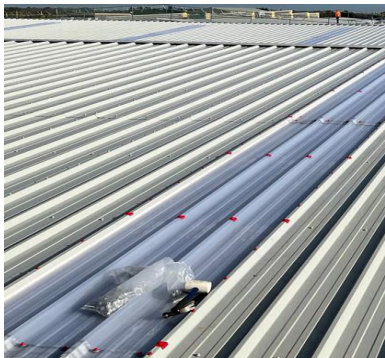
3.5 Roof Type 01 to include canopies— Trapezoidal profile in Goosewing Grey
