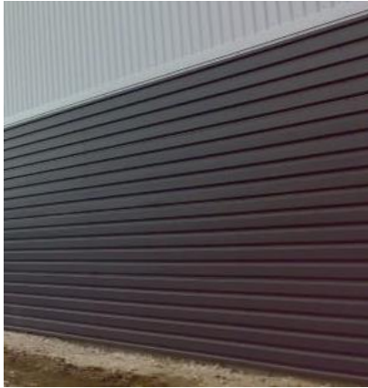
3.1 Trapezoidal profile, horizontally laid in Anthracite (RAL 7016)
