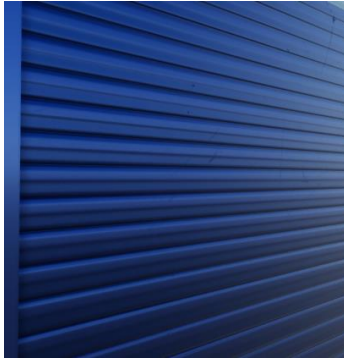
3.12 Trapezoidal profile, horizontally laid in Midnight Blue
