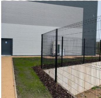
3.13 2.4m high Paladin Fencing
