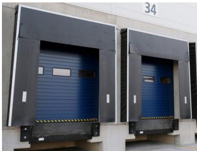
3.8 (B) Operational Door – Dock Door, sectional, insulated door Plastisol Coated Finish in Midnight Blue (RAL 5003)
