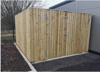
3.18 Timber-faced Bin Store enclosure
