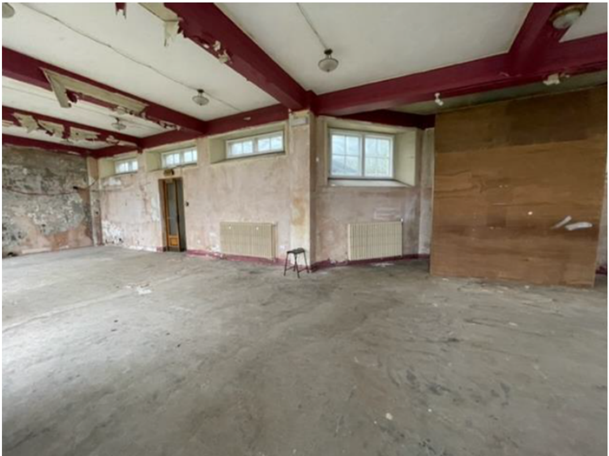
Existing interior facing entrance to toilet block
