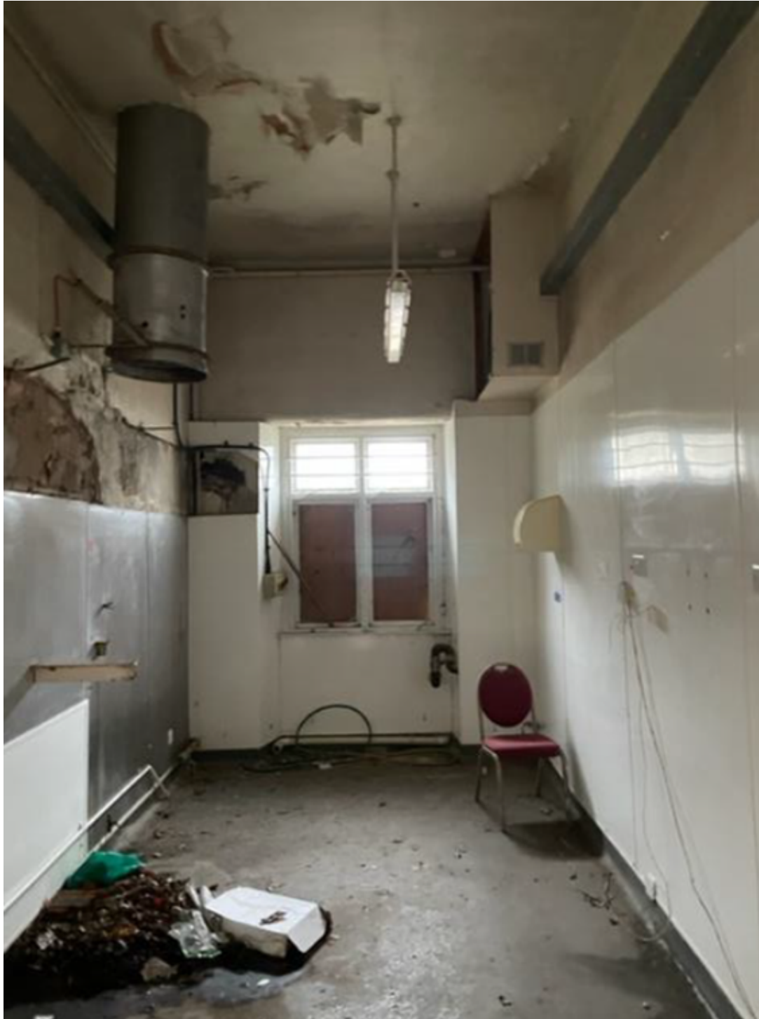
Former kitchen area
