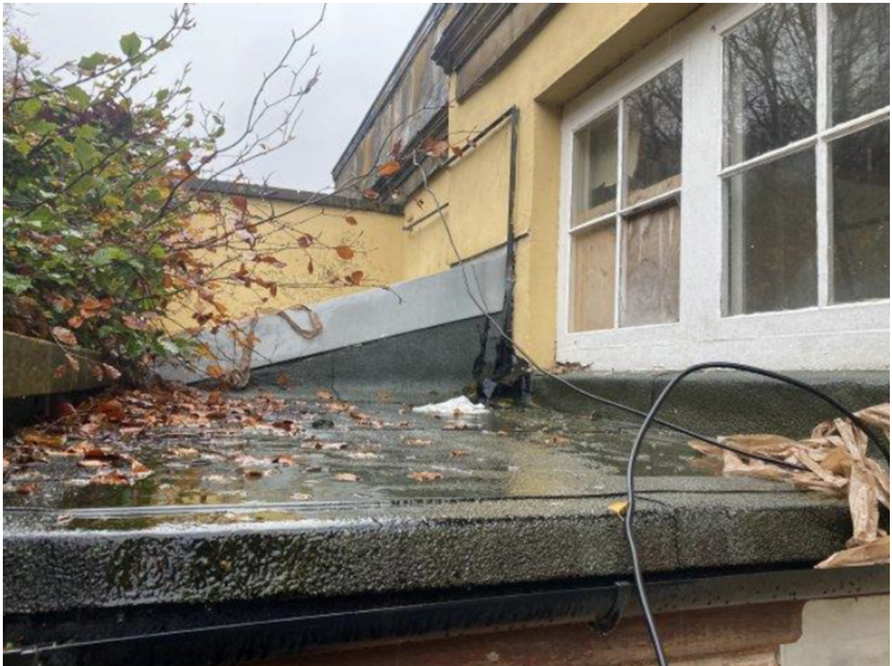
Window overlooking boiler room roof
