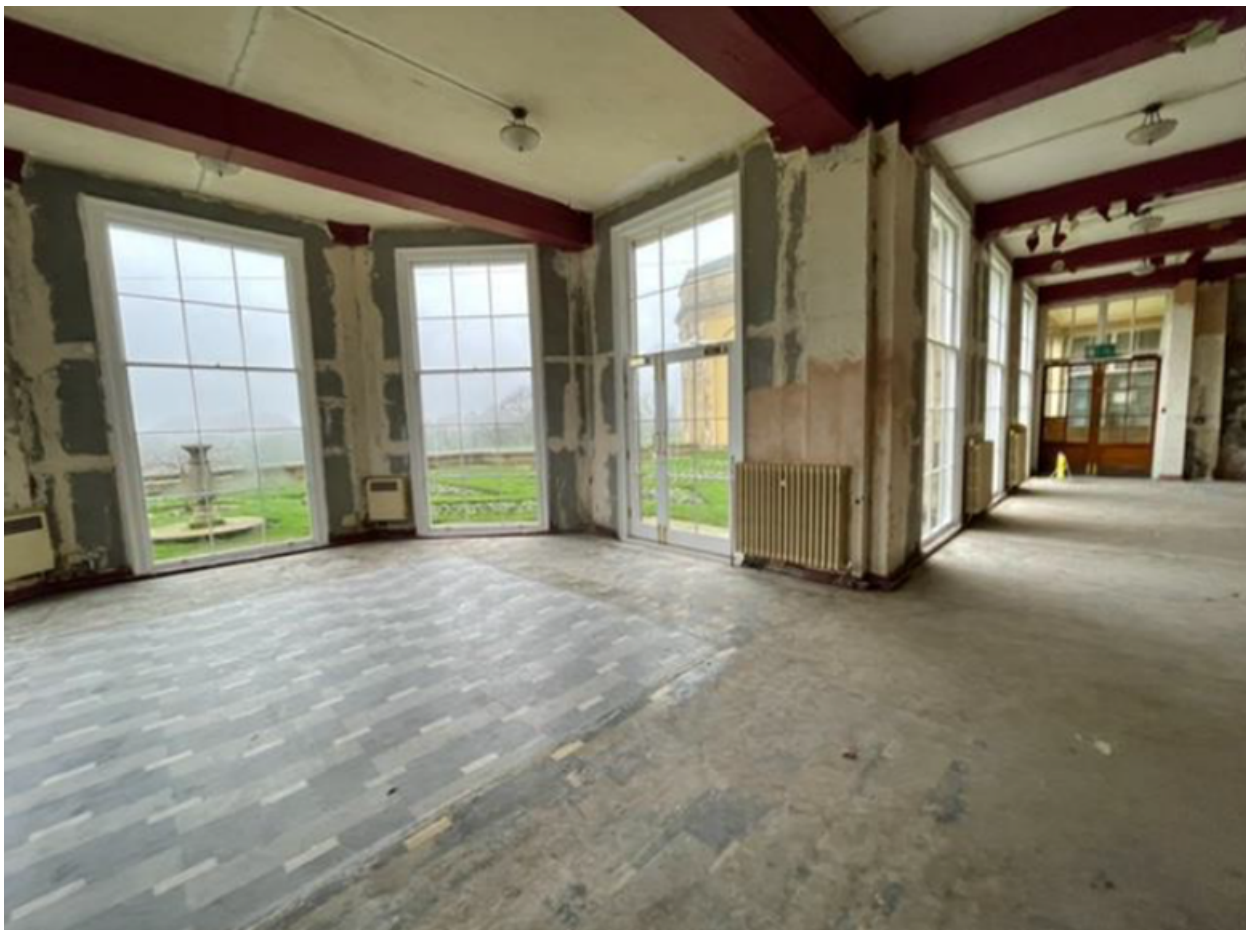
Existing interior facing west towards bay windows
