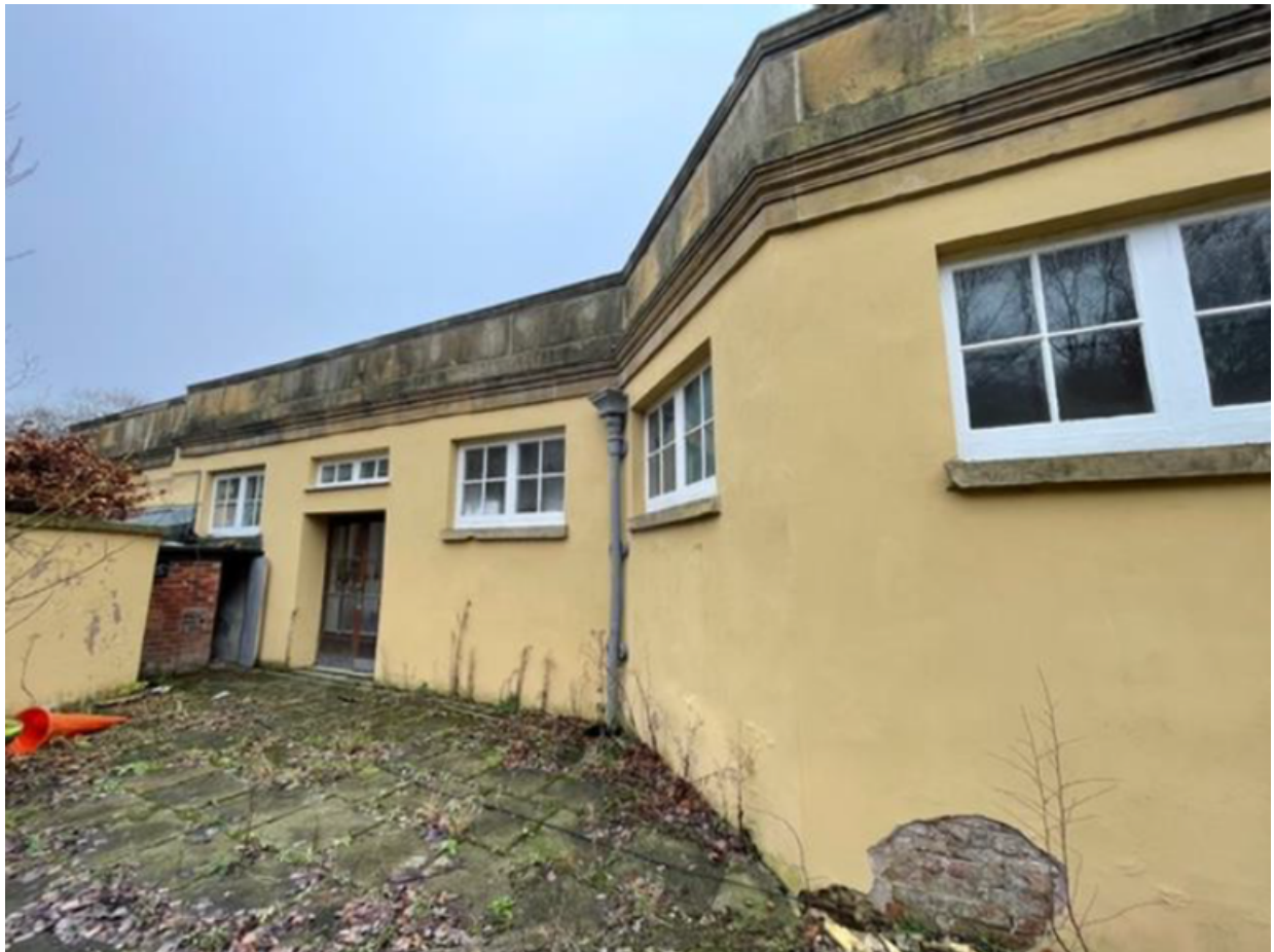
Existing courtyard elevation to rear of Orangery
