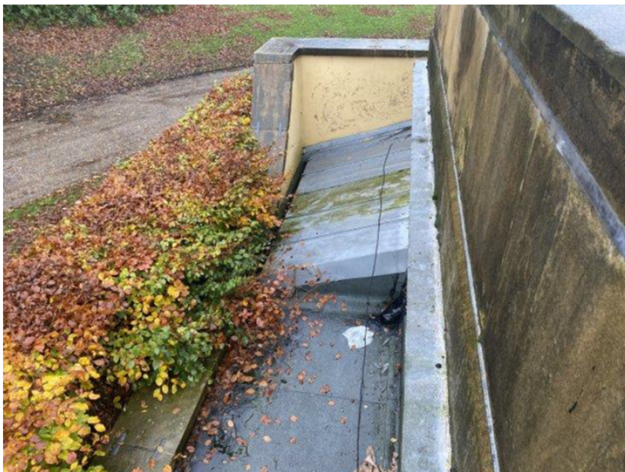
Rear entrance roof and boiler room roof
