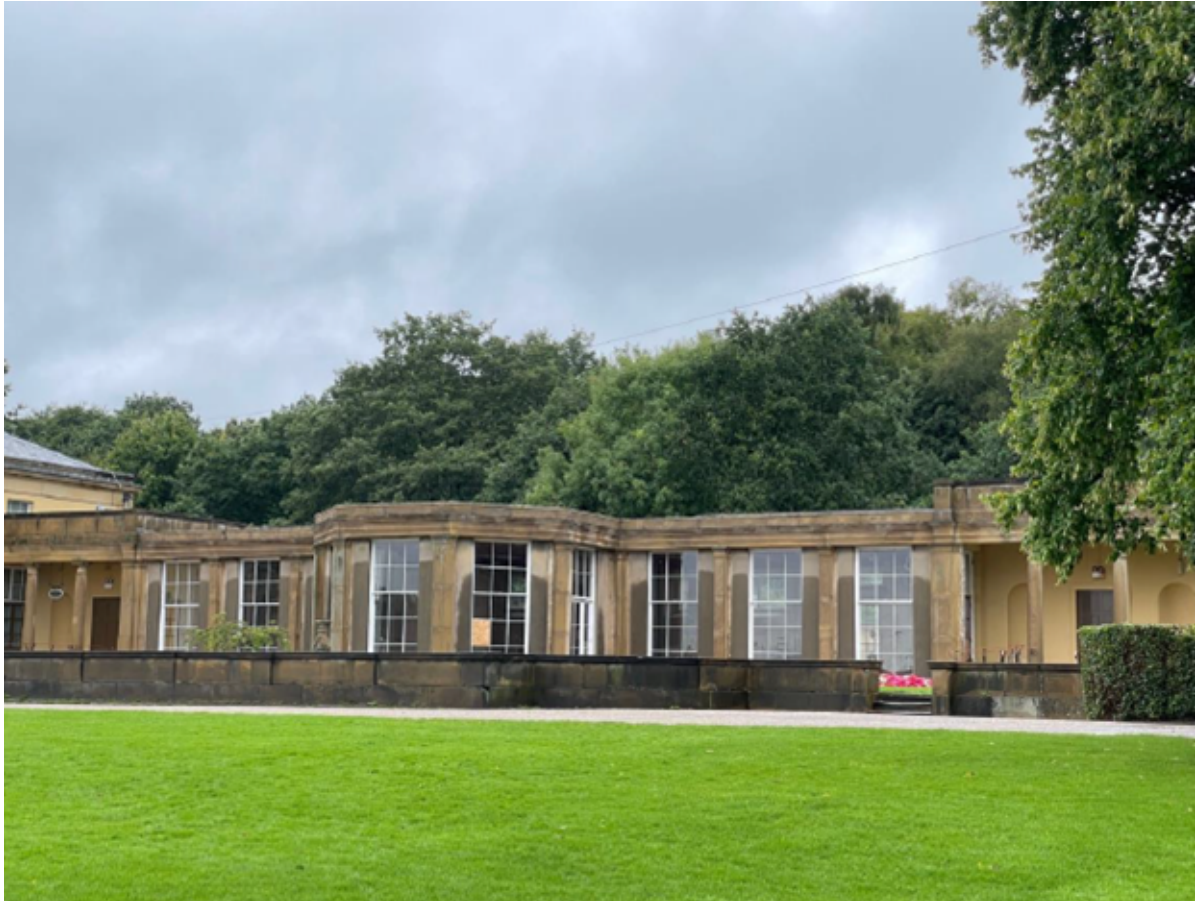
South facing elevation to the park
