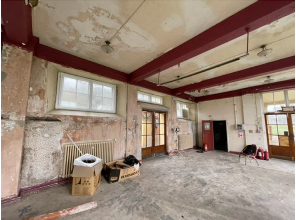
Existing interior facing towards proposed servery area
