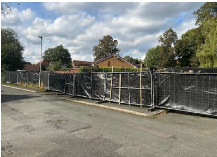
View from Grant Close looking west
