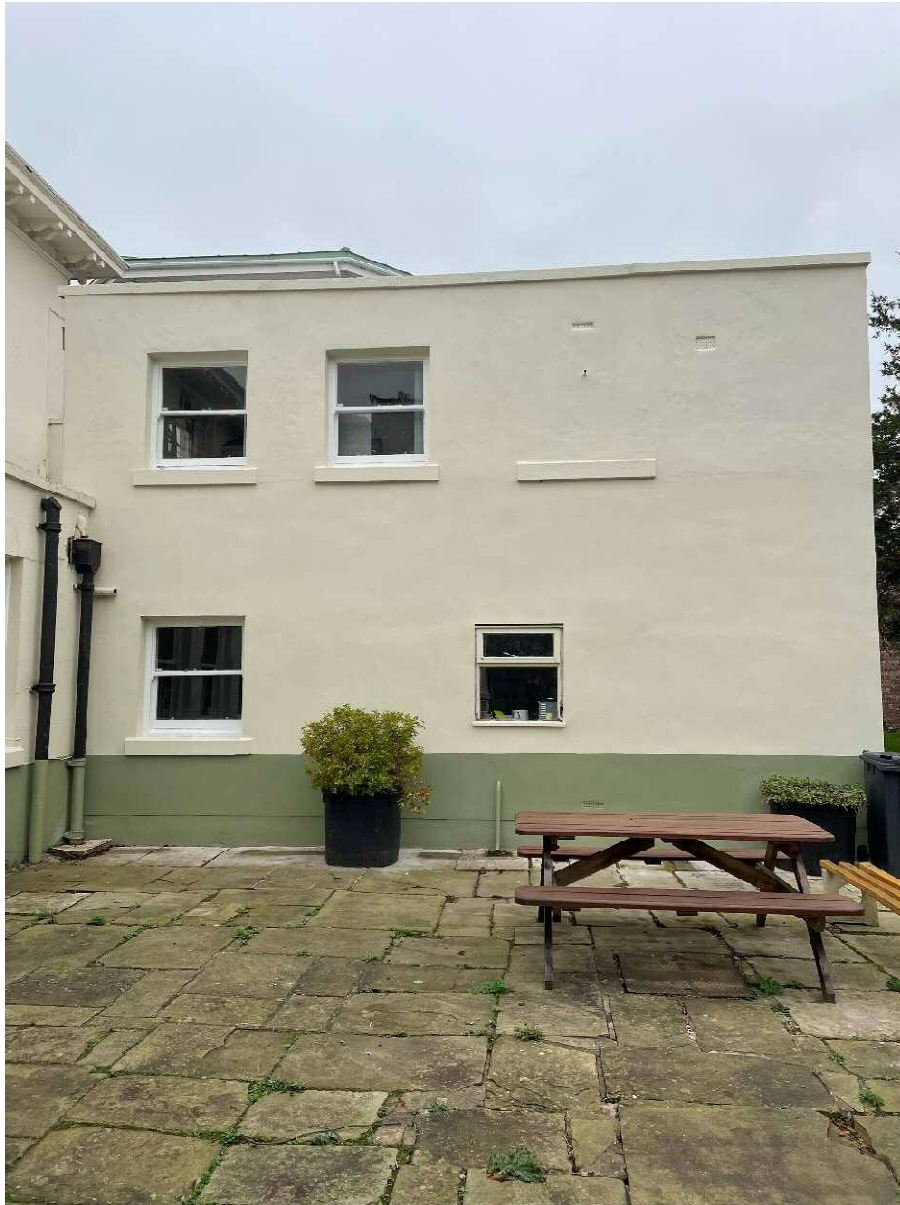
Photo 1. North elevation of St John's Annexe. Window to be replaced is the casement window to the right-hand side.
