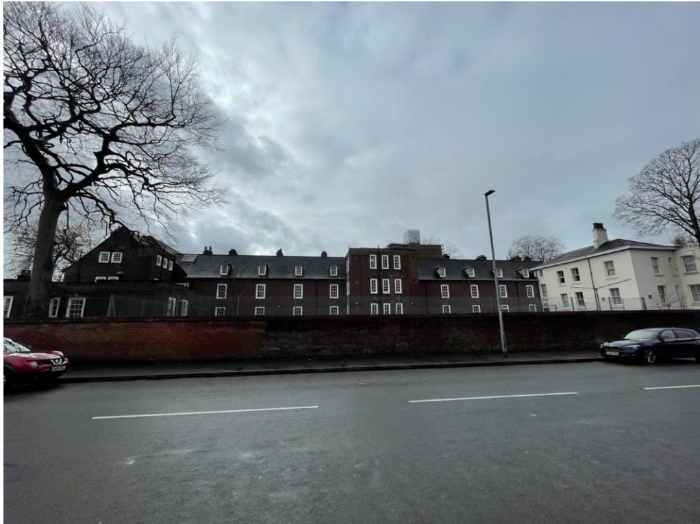
Figure 4.5: View of the Lees Wing of Ashburne Hall from the north on Old Hall Lane.
