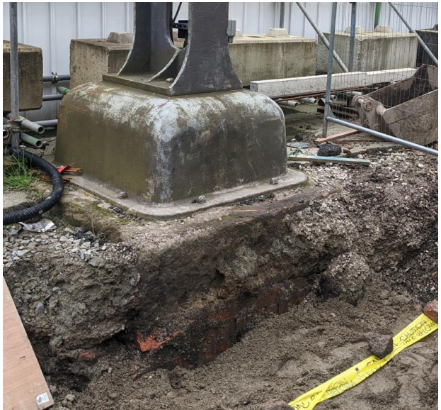
Figure 2-9 Plinth / foundation detail
