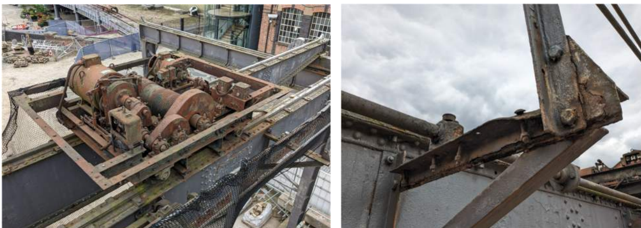
Figure 3-5 Craneage assembly (L) and balustrade support (R)
