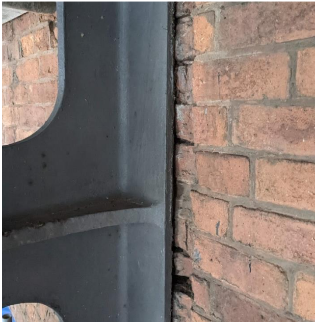
Figure 2-12 Power Hall interface
