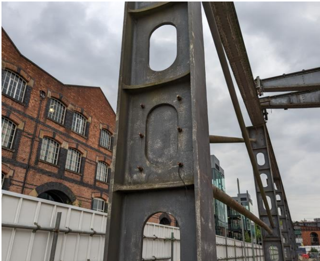
Figure 2-20 – North bracing connection detail
