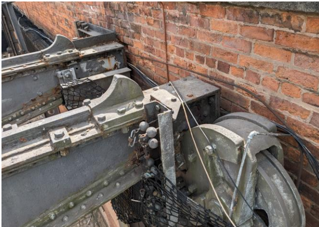
Figure 2-21 – Crane beam support
