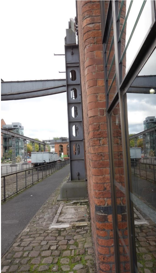
Figure 2-13 Power Hall interface
