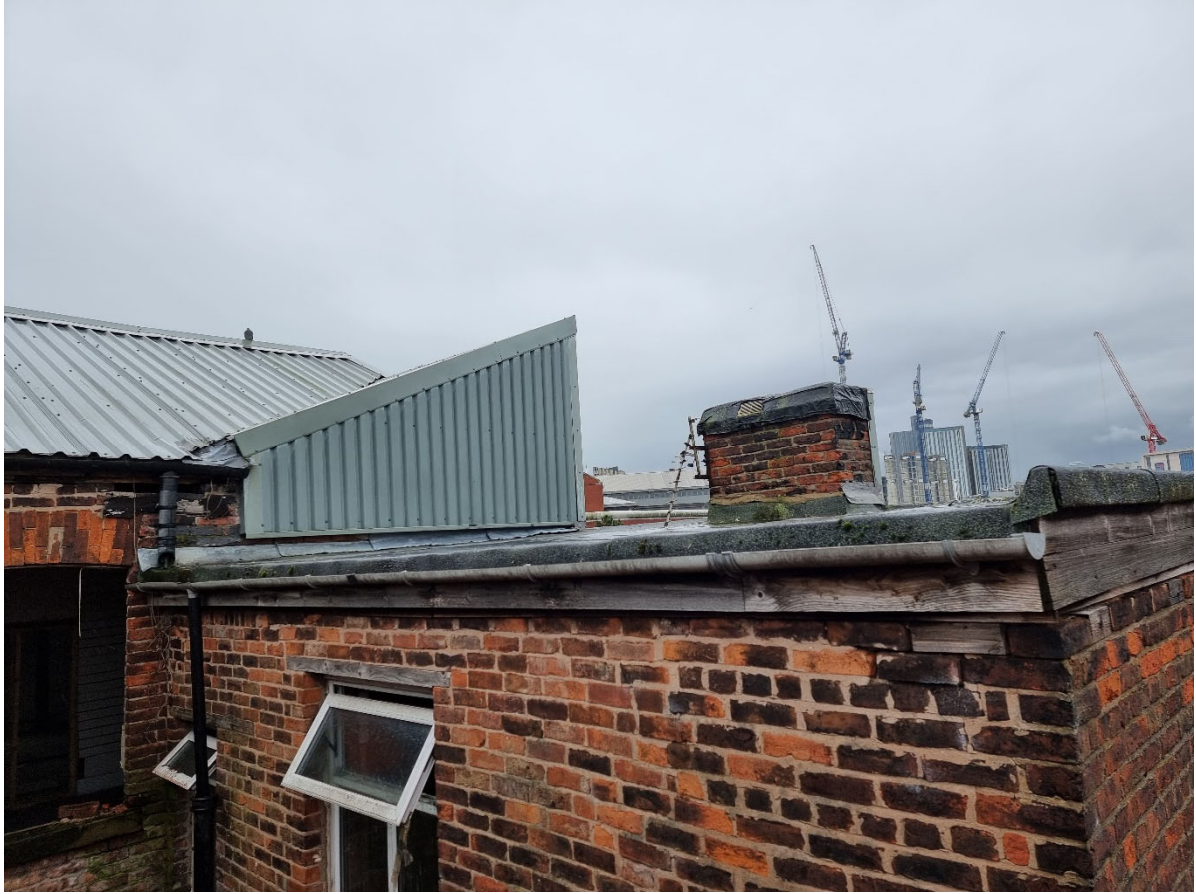
View of existing flat and pitched roofs to rear, above which proposed dormer to be constructed
