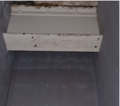
Existing cast iron beam visible in ceiling void above, to be exposed.
