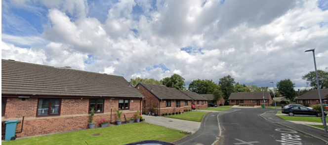
Above: Bungalows that are located on Thorntree Close which is located next to the site (North West)
