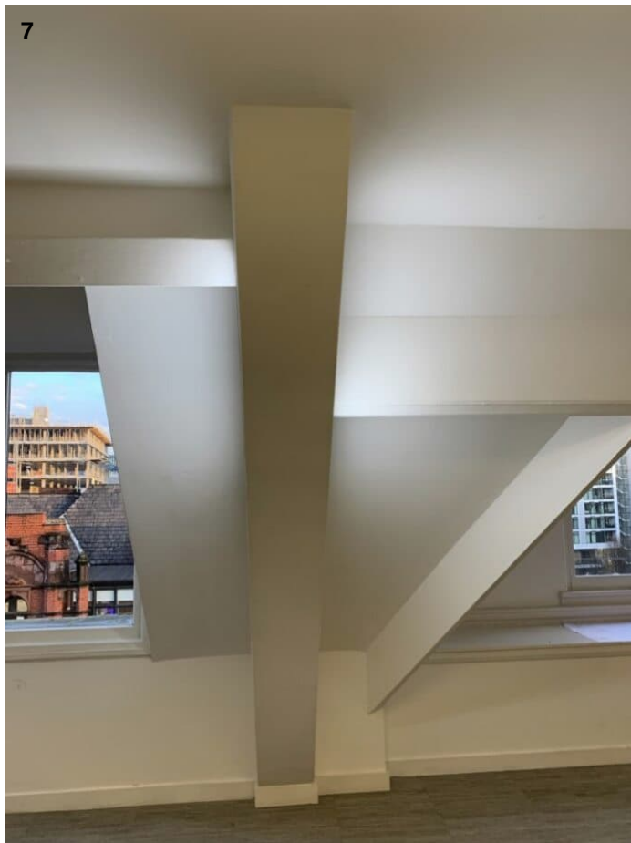
Timber beams to mansard roof
