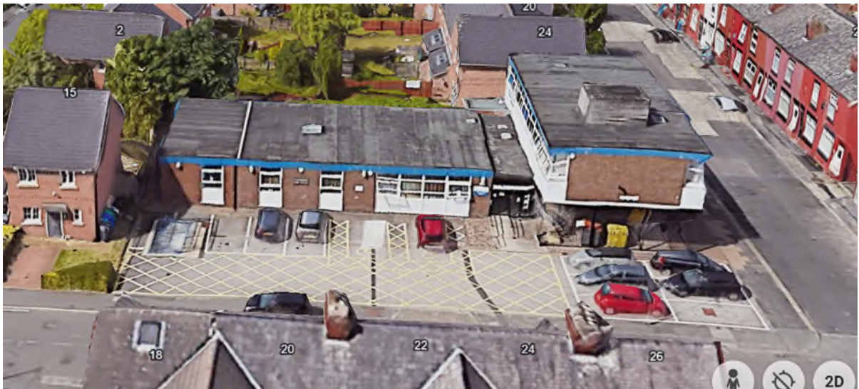
Aerial view of building
