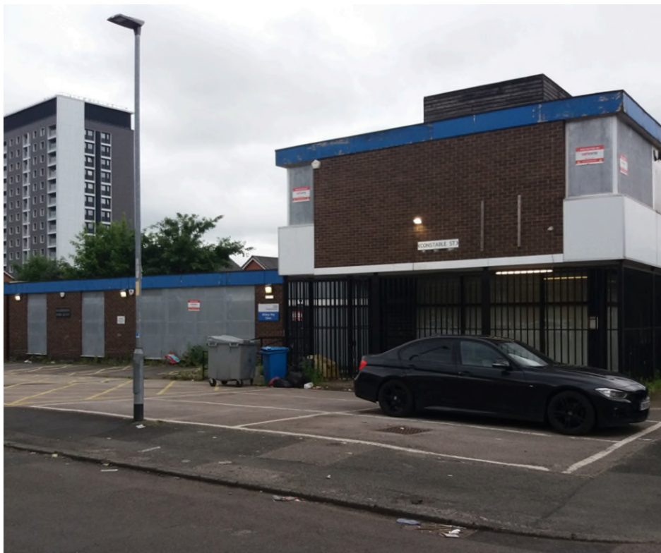
Existing building viewed from Constable Street
