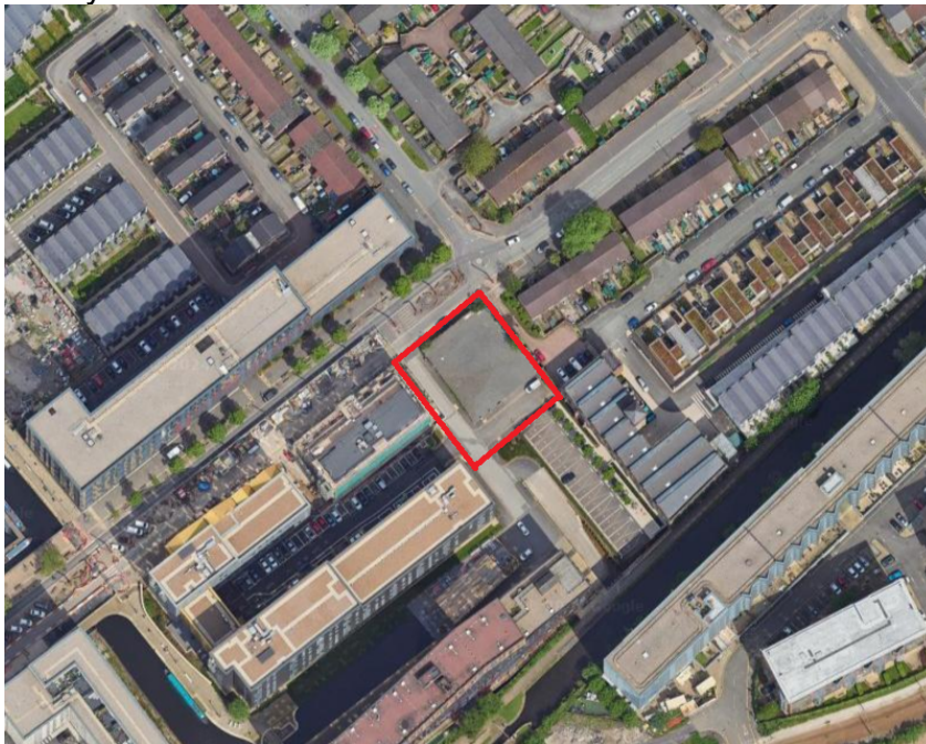
Aerial photograph of application site
