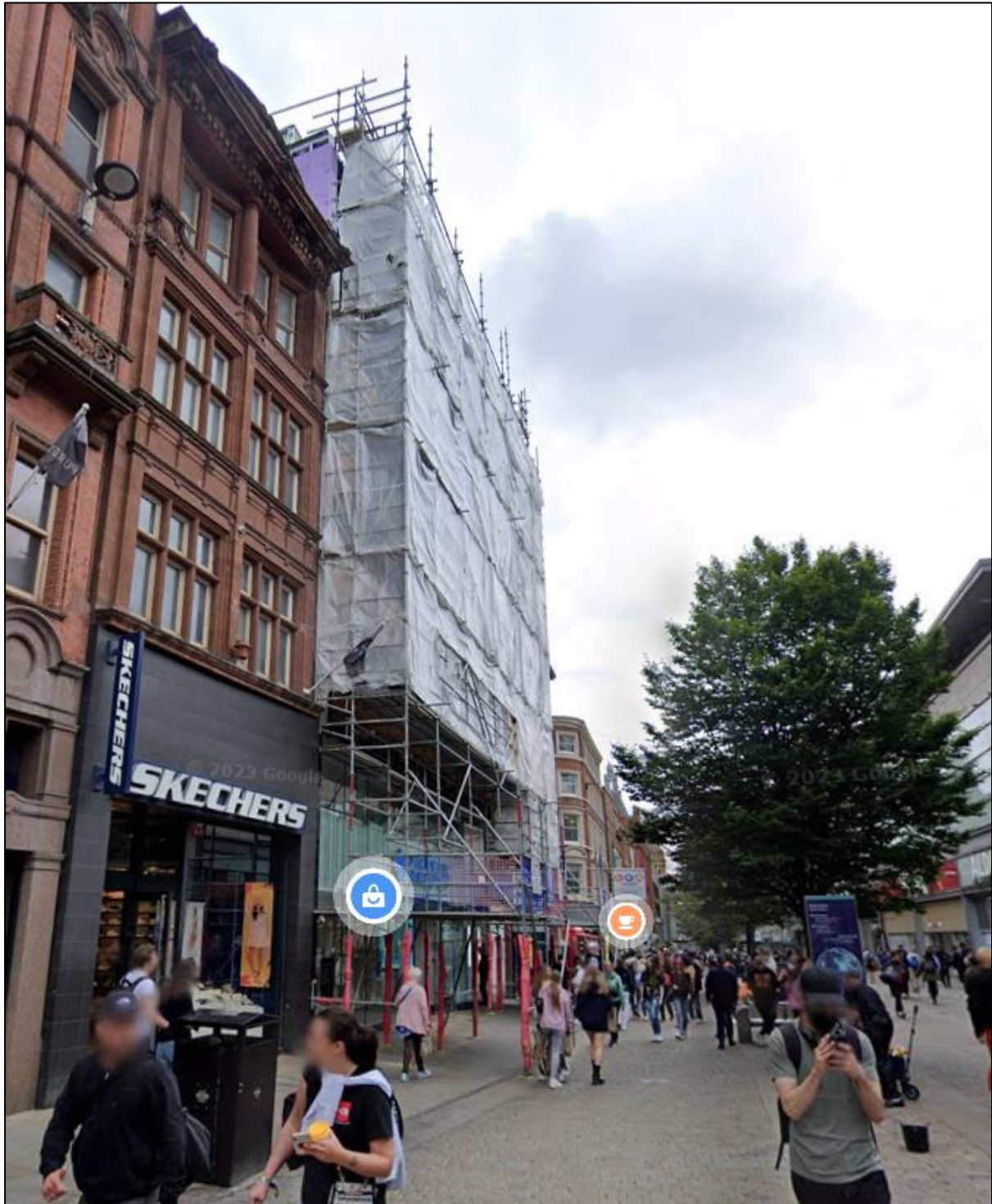
Fig 3: Example of negative visual impact of scaffolding on the street scene
