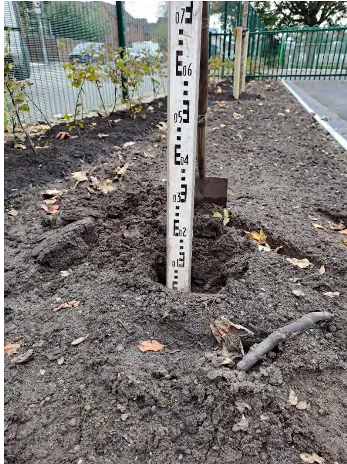
Plate 21: VP09 showing 200mm topsoil: Location Ornamental shrub and wildflower area adjacent to Reception Play Area.
