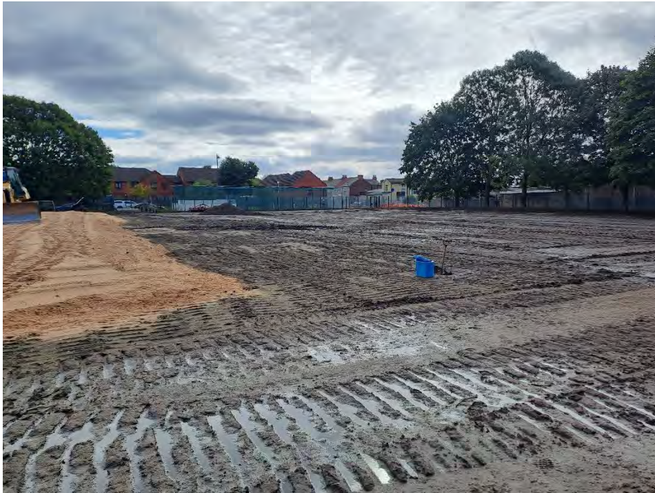
Plate 1: Topsoil laid over sports pitch with sand drainage layer being installed prior to turfing.
