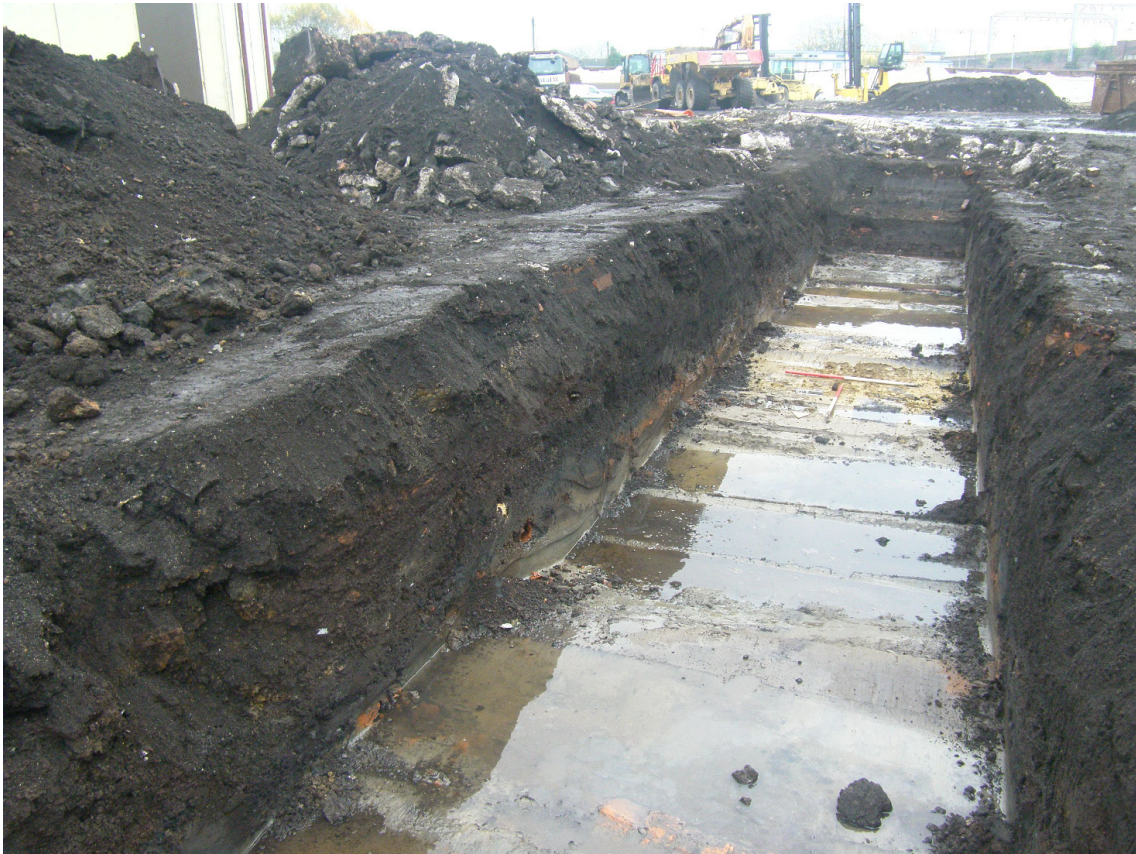
Plate 19 - Trench 8. Overview of trench, looking south-east
