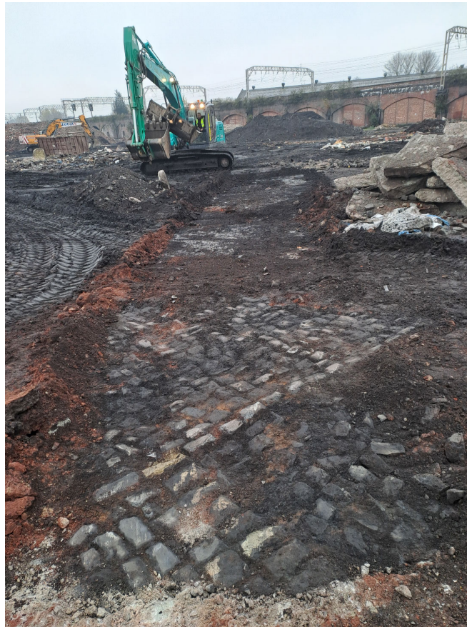
Plate 1 - Limestone setts in situ, overlying the location of Trench 2
