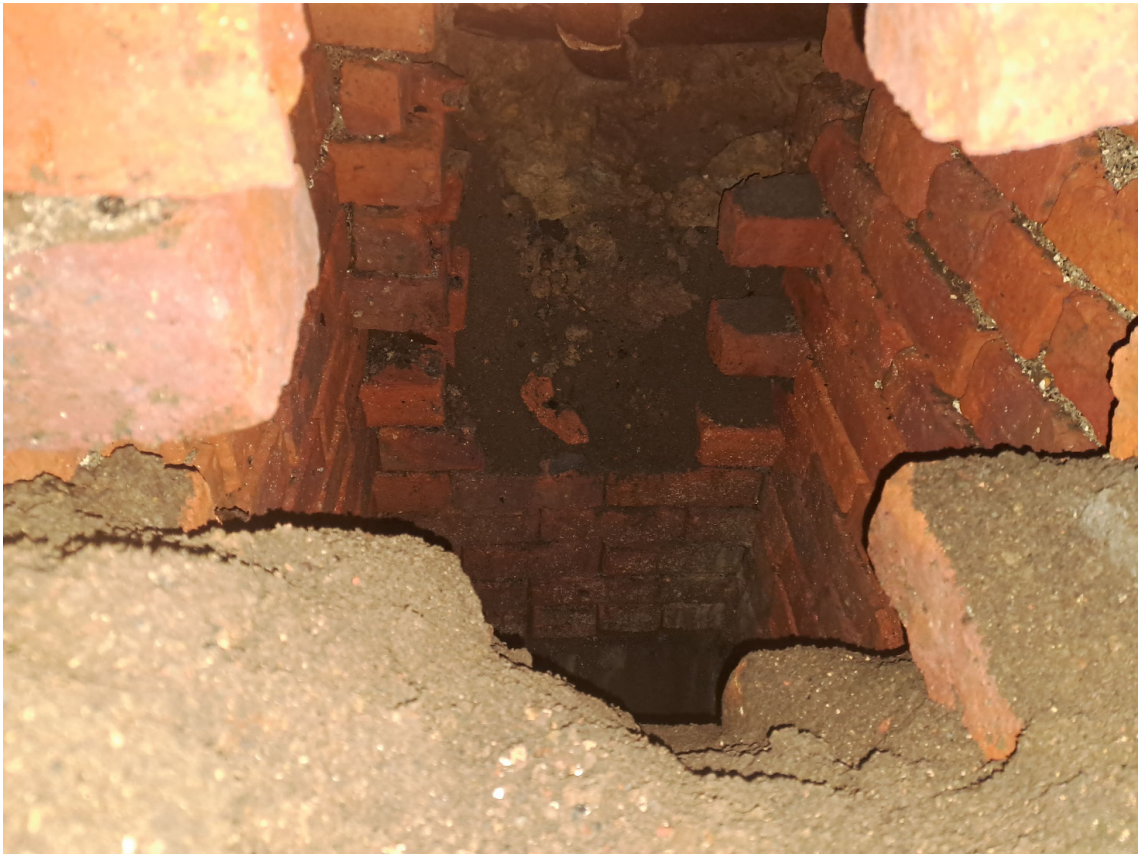
Plate 7 - Trench 2. Brick chute below platform 201
