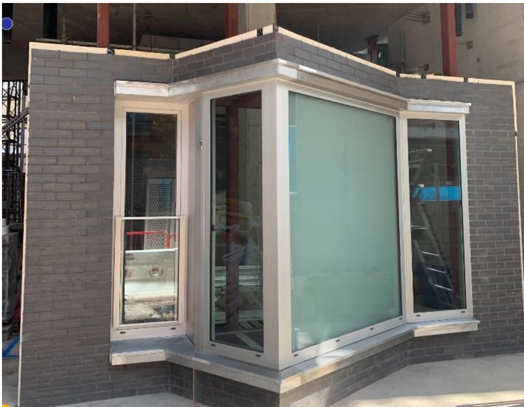
Sample panel 02: Sawtooth bay details
