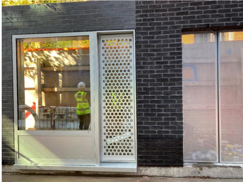
Sample panel 02: Sawtooth bay details
