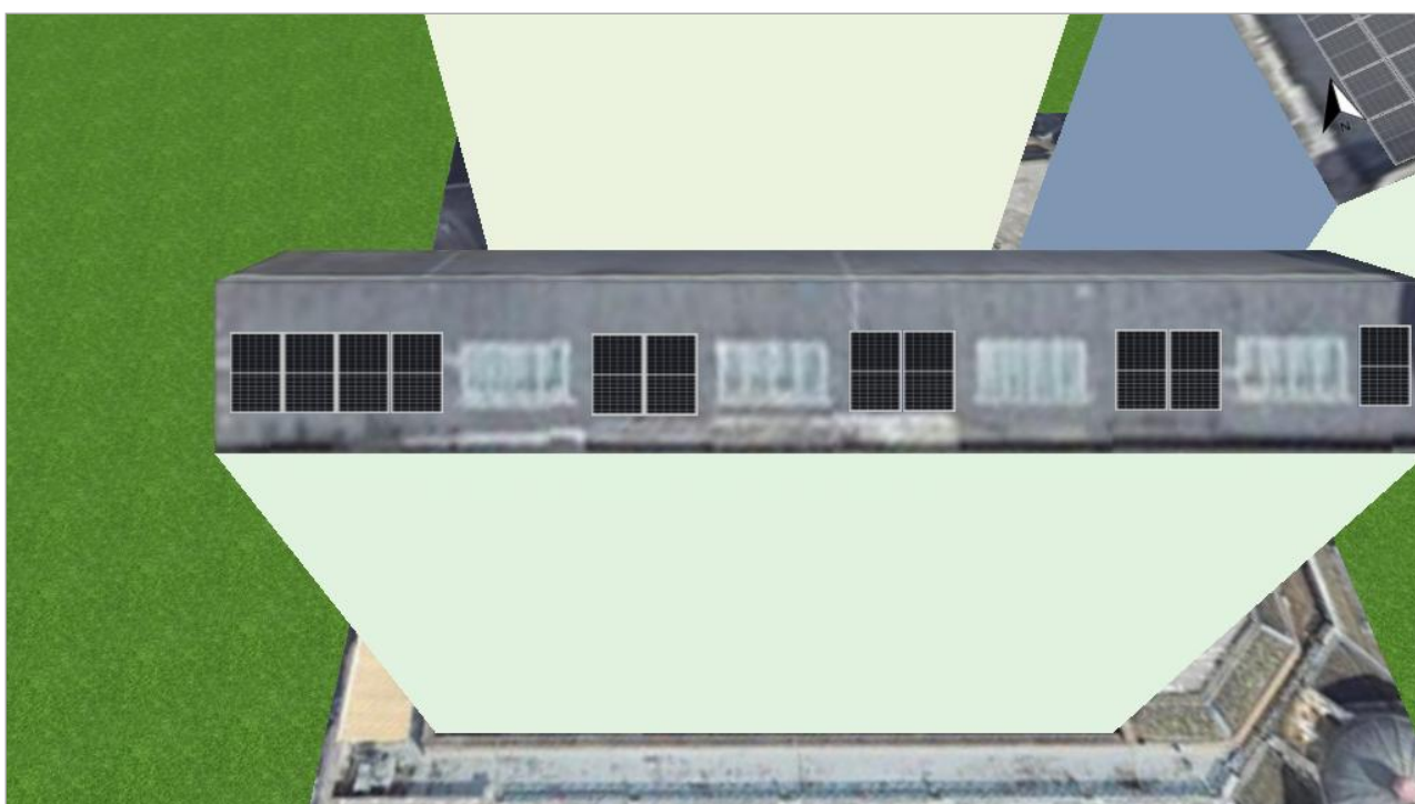
Figure: 1. Module Area - Building 01-Roof Area South
