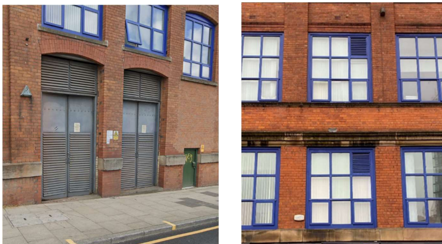
Figure 5.4 Existing louvred doors and louvred window panels at first and second floor
