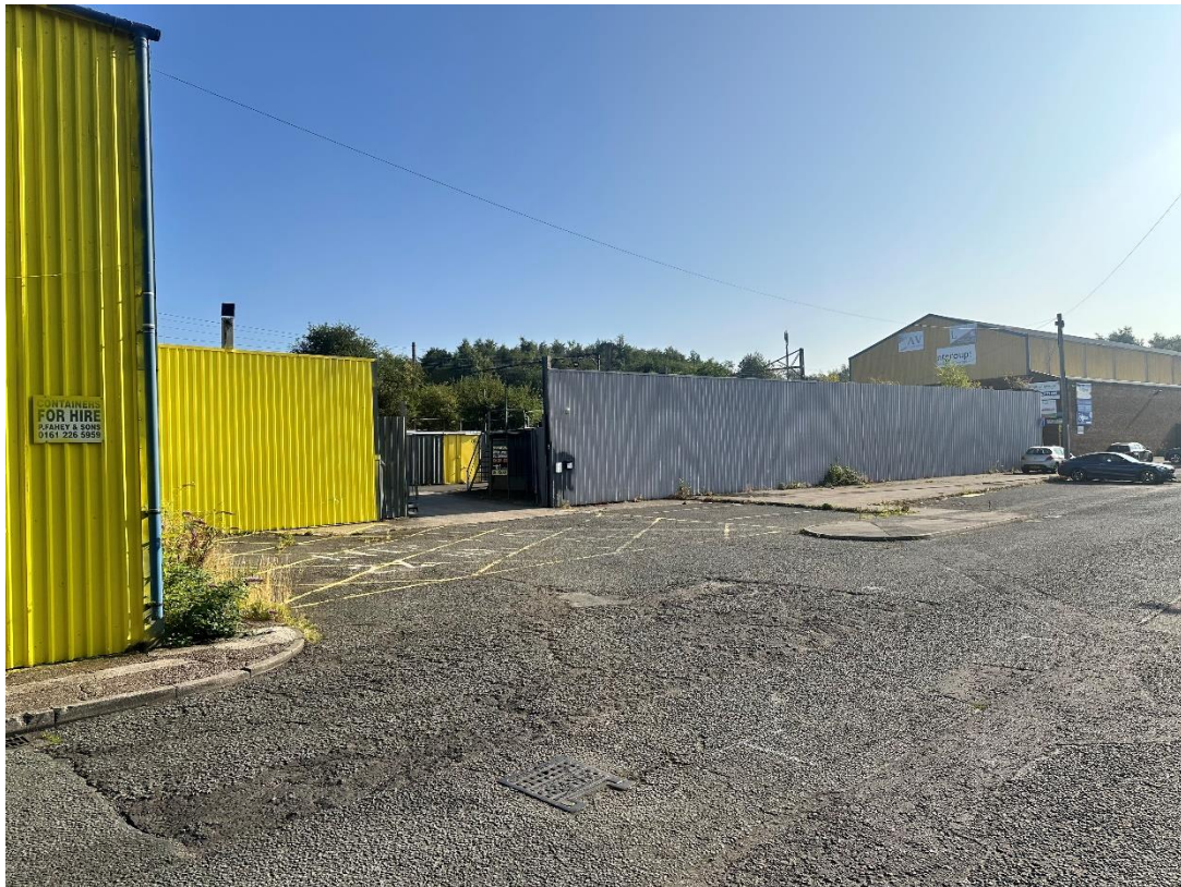
Entrance to adjacent site to the east
