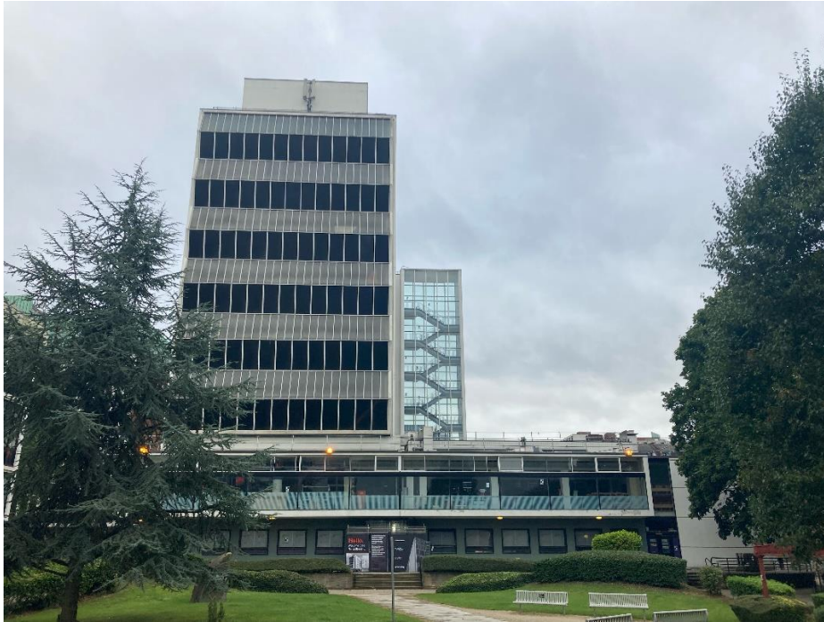
Figure 4- Before - View of Renold building from Courtyard before proposals
