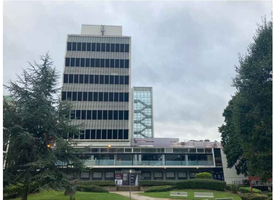
Figure 5- After - View of Renold building from Courtyard after proposals
