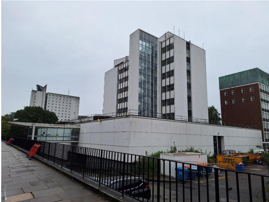
Figure 2- Before - View of Renold building from Altricham Street before proposals
