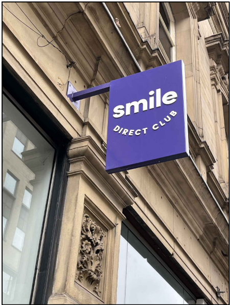
Photo reference: Existing blade sign fixing position to be retained
