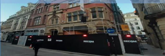
A view of the buildings that make up the application site from South King Street
