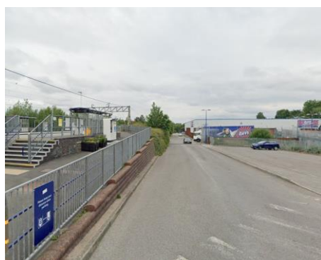
Site Rear – via Mauldeth Rd
