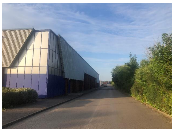
West Elevation & Access Road
