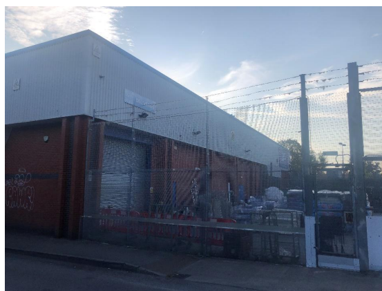
South Elevation and Loading Door
