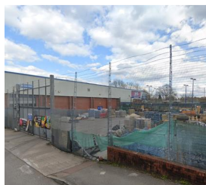
Site Rear – storage area
