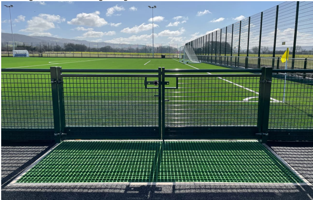
Double gate with in-fill mitigation grate:
