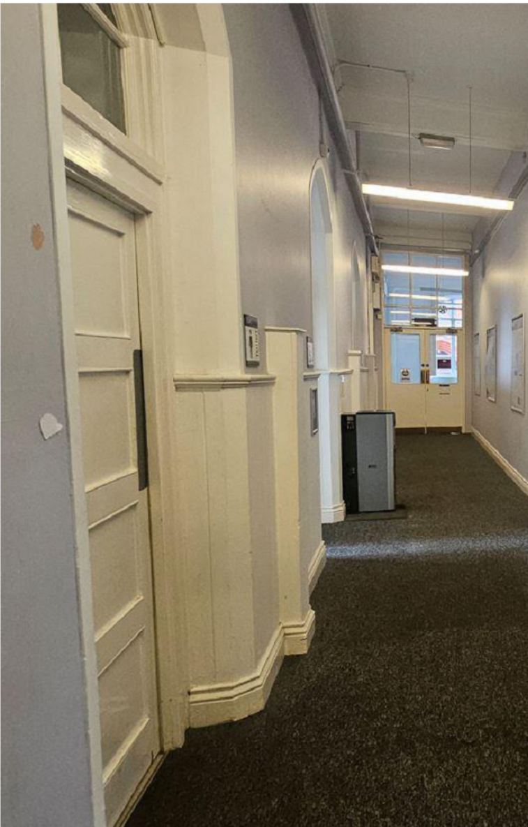
Existing doors opposite proposed EEG Lab along the corridor
