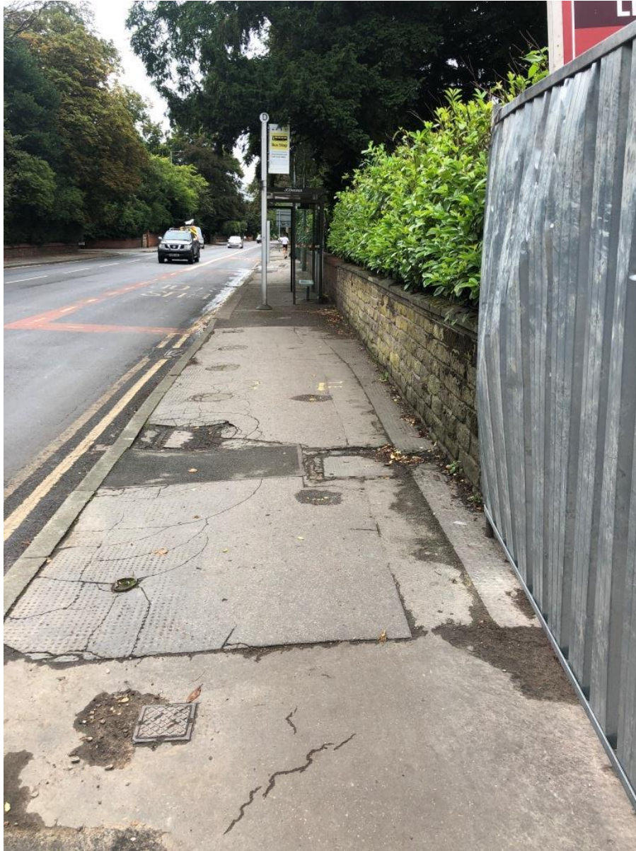
Fig. 5 – Secondary view showing footpath condition along the existing boundary wall.
