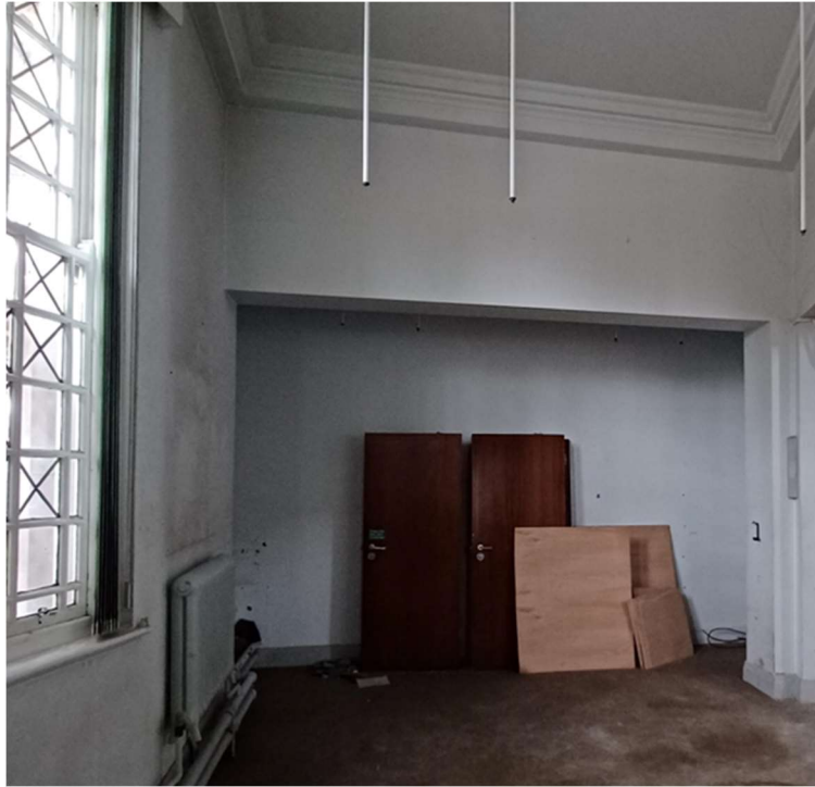
Partition wall as seen from within the staff room. Note the arch formed in the original wall.
