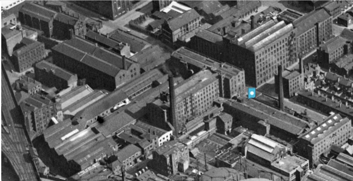
Figure 6 https://www.britainfromabove.org.uk/en/image/EPW062710 EPW062710 ENGLAND (1939). The Gaythorn Gas Works, Manchester, 1939
