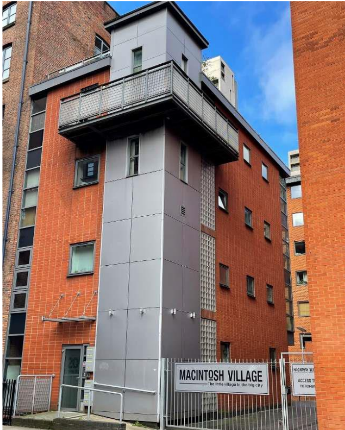
Figure 2 Photograph of the cladding to be replaced
